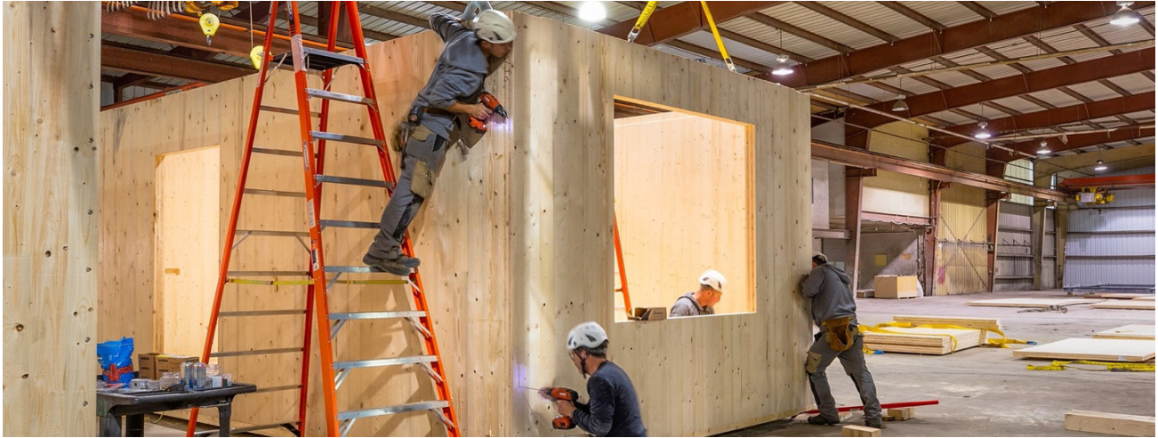
FIGURE 1: THE FORTERRA MODULAR CLT PROTOTYPE 2022 IS AN EXAMPLE OF MASS TIMBER PRODUCTS EVOLVING INTO MASS TIMBER SYSTEMS
