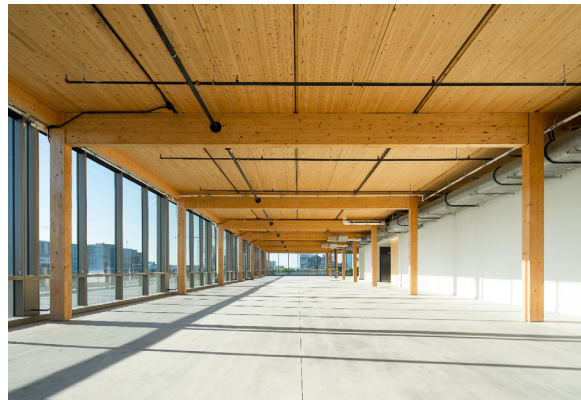
FIGURE 3: INHERENTLY, 2-BY-8 DLT HAS A 38 SOUND TRANSMISSION CLASS (STC) RATING. BUT WITH THE ADDITION OF A ¾-INCH ACOUSTI-MAT AND 3-INCH TOPPING SLAB, THE STC CAN EXCEED 50. THAT HELPS MITIGATE NOISE FROM ABOVE AND FORMS A CREATIVE SPACE FOR SINGERS AND SONGWRITERS.
