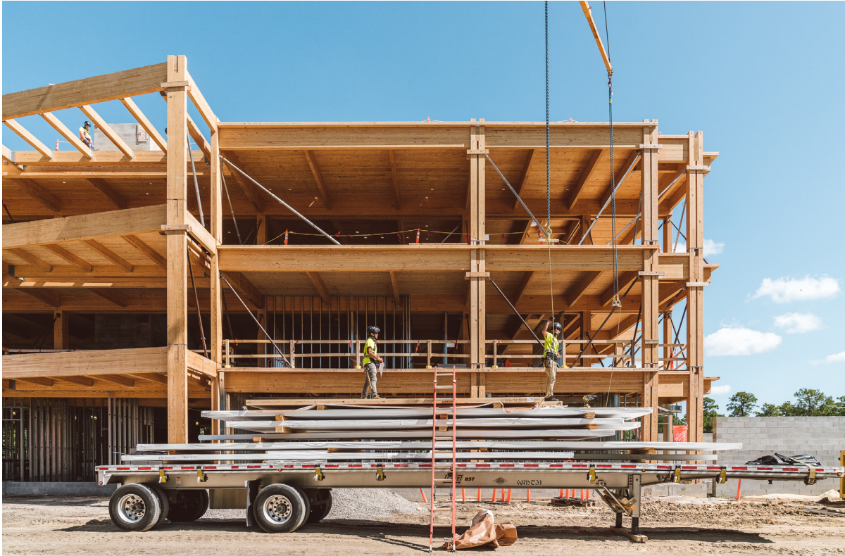
MASS TIMBER DELIVERY AND INSTALLATION
