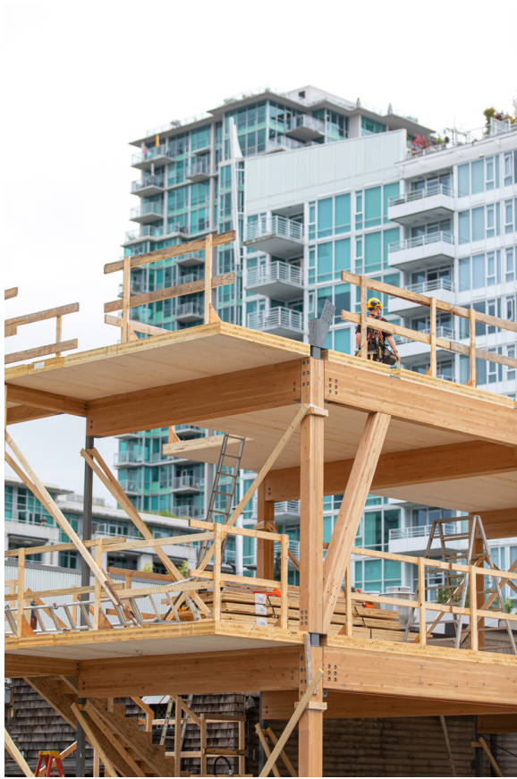
CONSTRUCTION OF 1 LONSDALE AVENUE PROJECT IN NORTH VANCOUVER, BC
