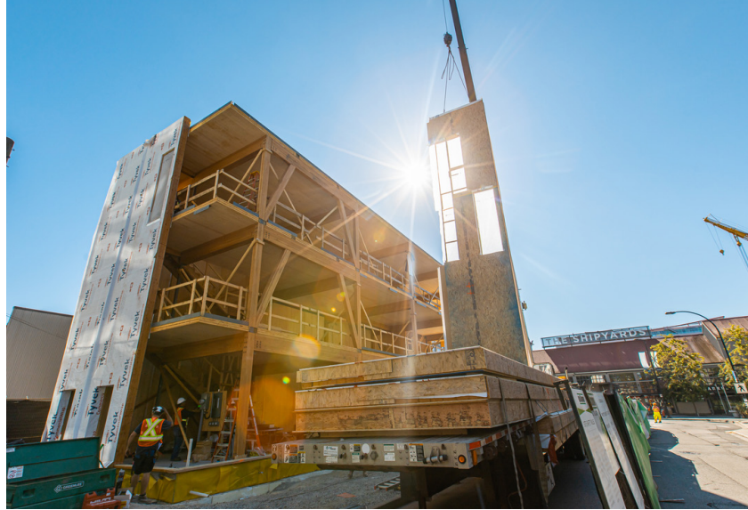
CLT PANEL DELIVERY AT 1 LONSDALE AVENUE PROJECT IN NORTH VANCOUVER, BC
