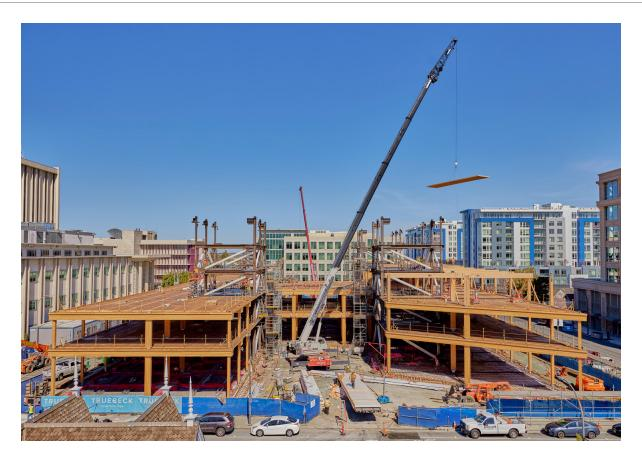
**THE MASS TIMBER FRAME IS ERECTED AT SAN MATEO COUNTY'S COB3.** Source: Truebeck Construction; Credit: Cesar Rubio
