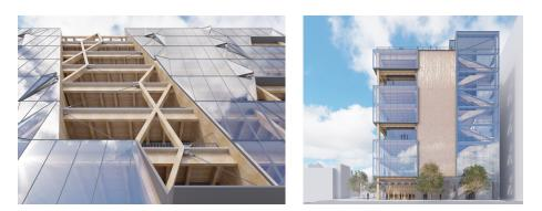
LEFT — WITH A MULTITUDE OF OPERABLE WINDOWS AND OUTDOOR SPACES, THE WORKPLACE PORTION OF THE FLOOR WILL HAVE ABUNDANT ACCESS TO FRESH AIR. RIGHT — FLIPPING THE FIRE STAIR TO THE PERIMETER NOT ONLY FLOODS IT WITH DAYLIGHT AND AMENABLE VIEWS BUT ALSO TRANSFORMS IT INTO A MULTIUSE TENANT AMENITY. Source: Gensler
