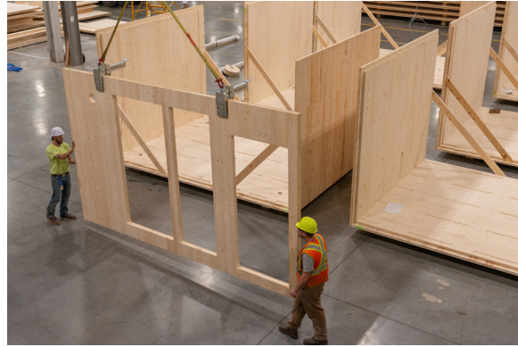
WORKERS ASSEMBLE GREEN CANOPY NODE'S MASS TIMBER MODEL HOME.
