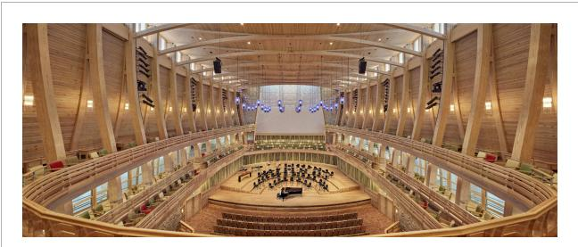
CAPTURING THE ESSENCE OF THE CONCERT HALL: 'TUNING FORK' COLUMNS HARMONIZING WITH HYBRID TRUSSES AND A CONVEX TIMBER DECKING CEILING DESIGN
