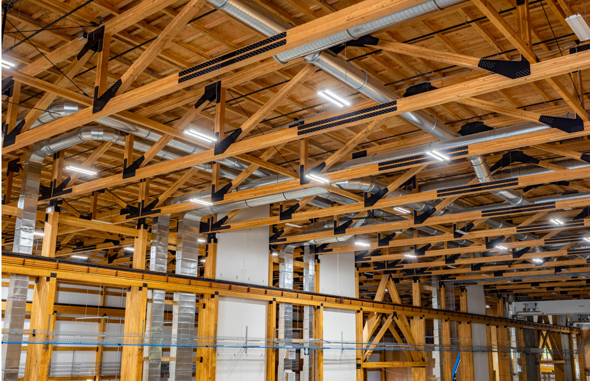
ONE HUNDRED-FOOT OPEN SPAN GLULAM TRUSS SYSTEM.
