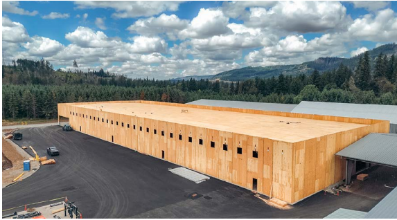
FRERES ENGINEERED WOOD'S PLYWOOD WAREHOUSE, BEFORE CLADDING
