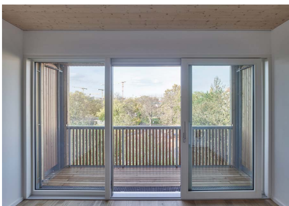
LEFT — CEILINGS WERE MADE OF VISUAL-QUALITY CLT
