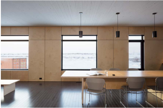
THE INTERIOR OF THE CENTRE WITH EXPOSED NAIL-LAMINATED TIMBER (NLT) CEILING
