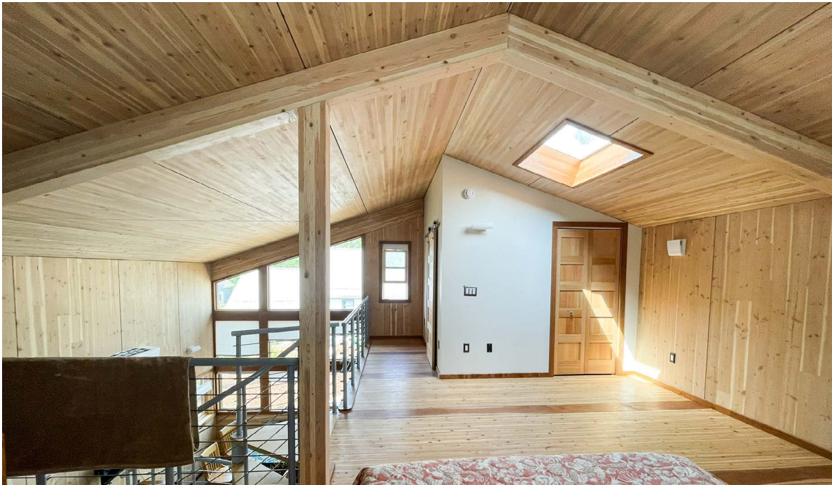
THE MƏXIṬP HOME IS CONSTRUCTED WITH CLT WALLS AND GLULAM ROOF AND FLOOR
