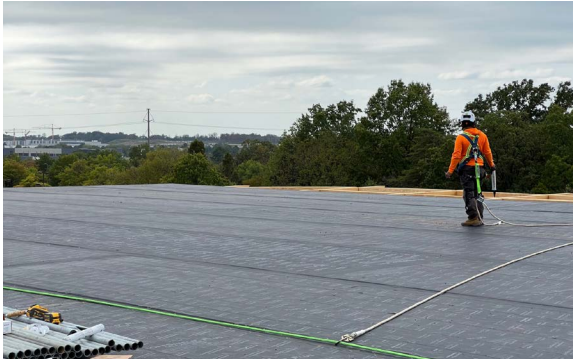
SLOPESHIELD PLUS ADHERED TO 3-PLY CLT PANELS
