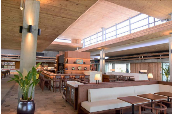
CLT PANELS INSIDE THE FINISHED AIRPORT
