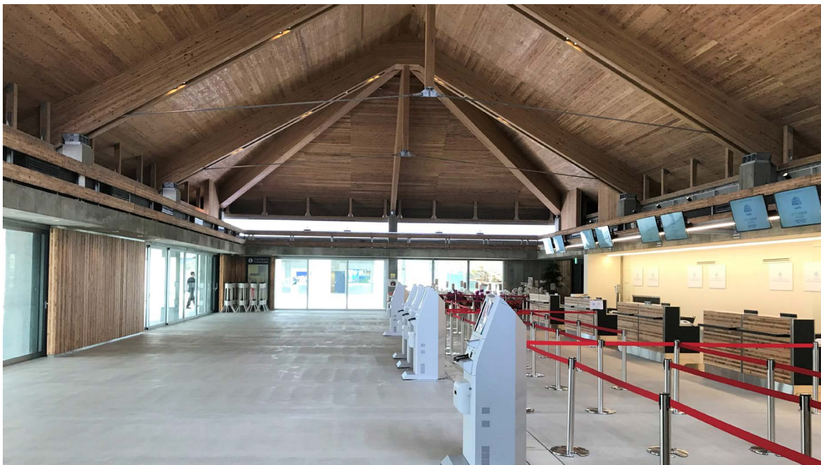
CLT PANELS THAT HAVE BEEN TREATED TO STAY FREE OF DECAY AND WOOD-DESTROYING ORGANISMS INSIDE FINISHED AIRPORT
