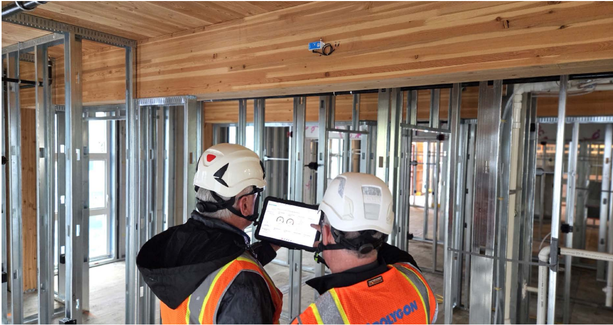
POLYGON SENSORS MONITOR WOOD MOISTURE CONTENT ON TRUEBECK'S MASS TIMBER PROJECT
