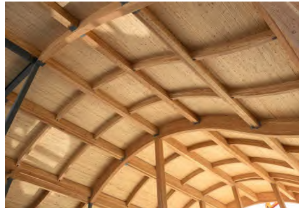
THE CURVED CEILINGS IN THE BRIGHTWATER BUILDING IN PORT CREDIT, ONTARIO, SHOWCASE THE DESIGN FLEXIBILITY OFFERED BY NLT PANELS
