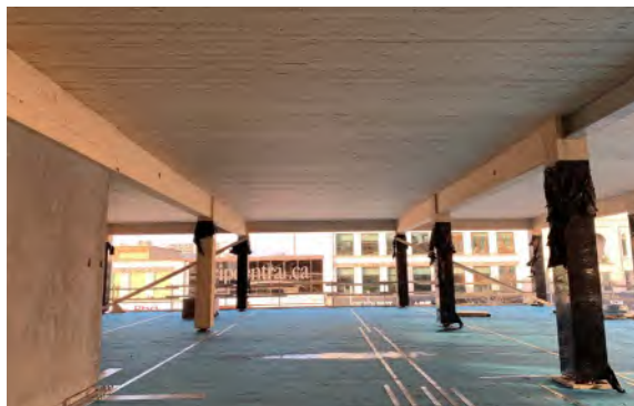
THE CEILINGS IN THE ONE YOUNG MASS TIMBER BUILDING IN KITCHENER, ONTARIO, FEATURE NLT PANELS THAT HIGHLIGHT THE STRENGTH, SUSTAINABILITY, AND NATURAL BEAUTY OF ENGINEERED WOOD SOLUTIONS
