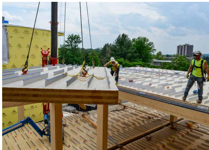
FIGURE 5.6 COMPOSITE CONCRETE-TIMBER SLABS WITH FLANGES 5
