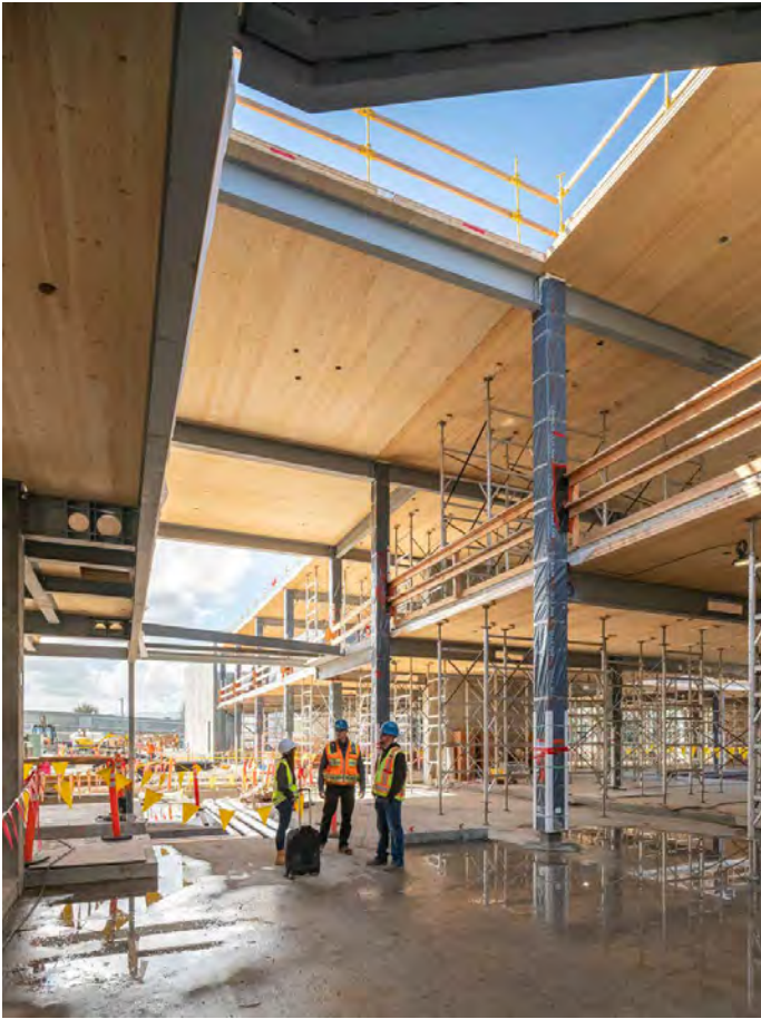
FIGURE 5.13 CONCRETE CORES AND PRECAST CONCRETE FRAME WITH TIMBER SLAB AND BEAMS. 13
