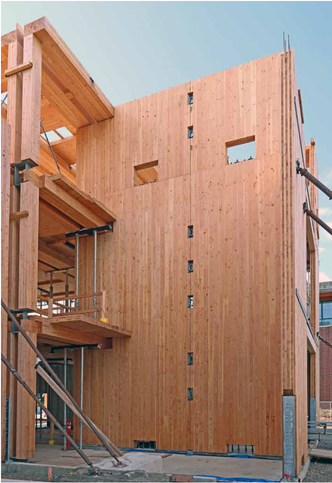
(LEFT) FIGURE 8.4 CLT POST-TENSIONED “ROCKING” SHEAR WALL 8
