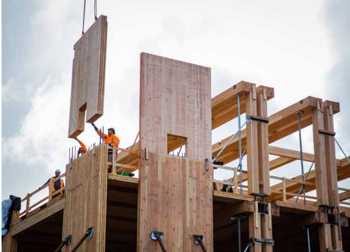
FIGURE 5.10 POST-TENSIONED CLT SHEAR WALL INSTALLATION 9
