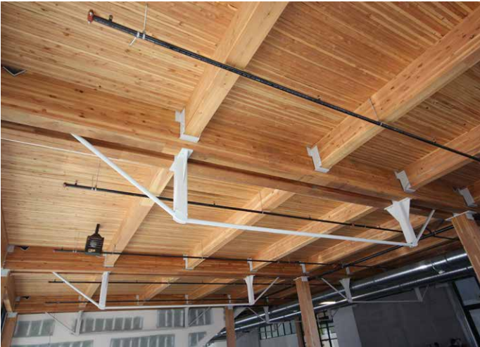
FIGURE 5.7 POST-TENSIONED TIMBER BEAM 6
