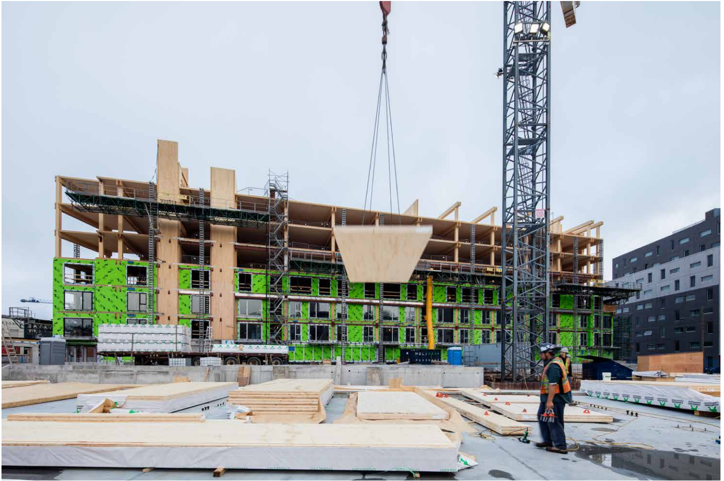
FIGURE 6.12 MASS TIMBER MATERIALS HANDLING 19
