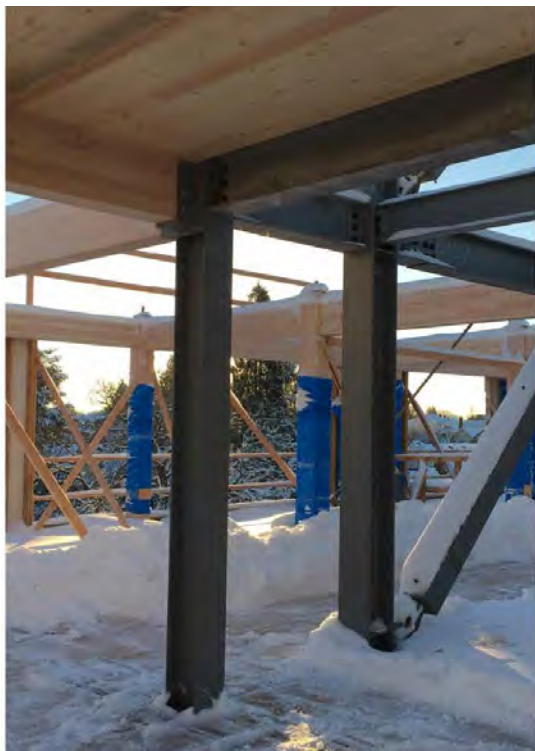
FIGURE 6.16 TIMBER FRAME AND STEEL CORE PROGRESSING IN COLD, SNOWY WEATHER 24
