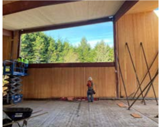
FIGURE 6.9: CLT WALL AND ROOF PANELS WITH STEEL FRAMING
