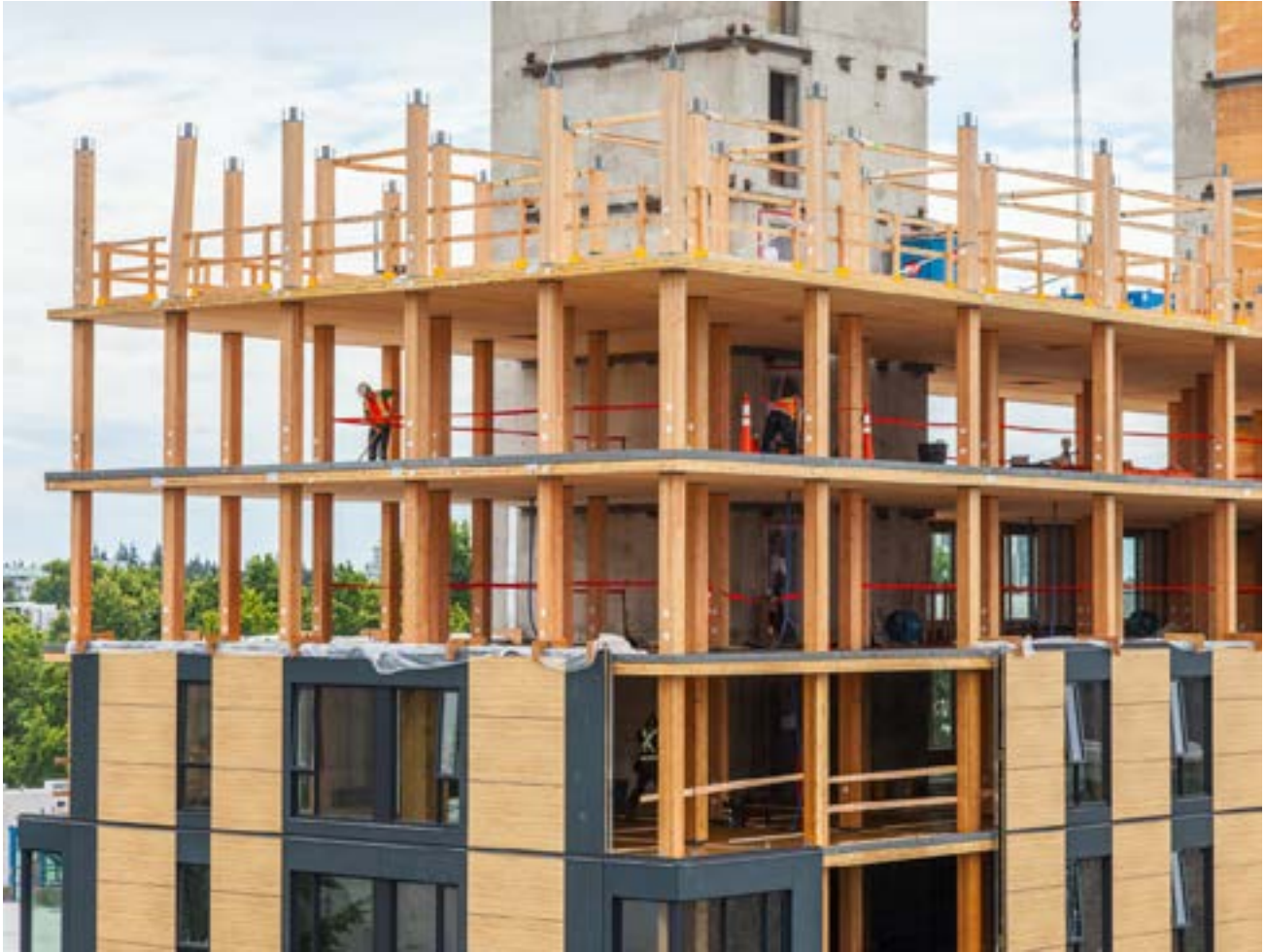
FIGURE 6.4: FACADE PANELS FOLLOW CLOSELY BEHIND STRUCTURAL FRAMING
