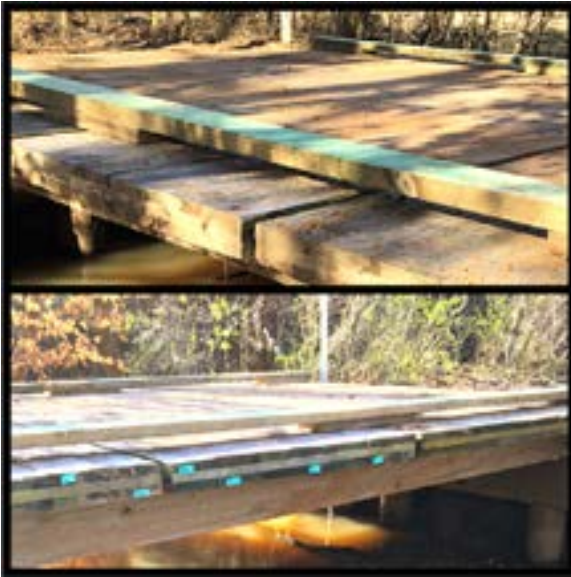
FIGURE 4.6: PRESERVATIVE-TREATED MASS TIMBER IN USE AS BRIDGE DECKING
