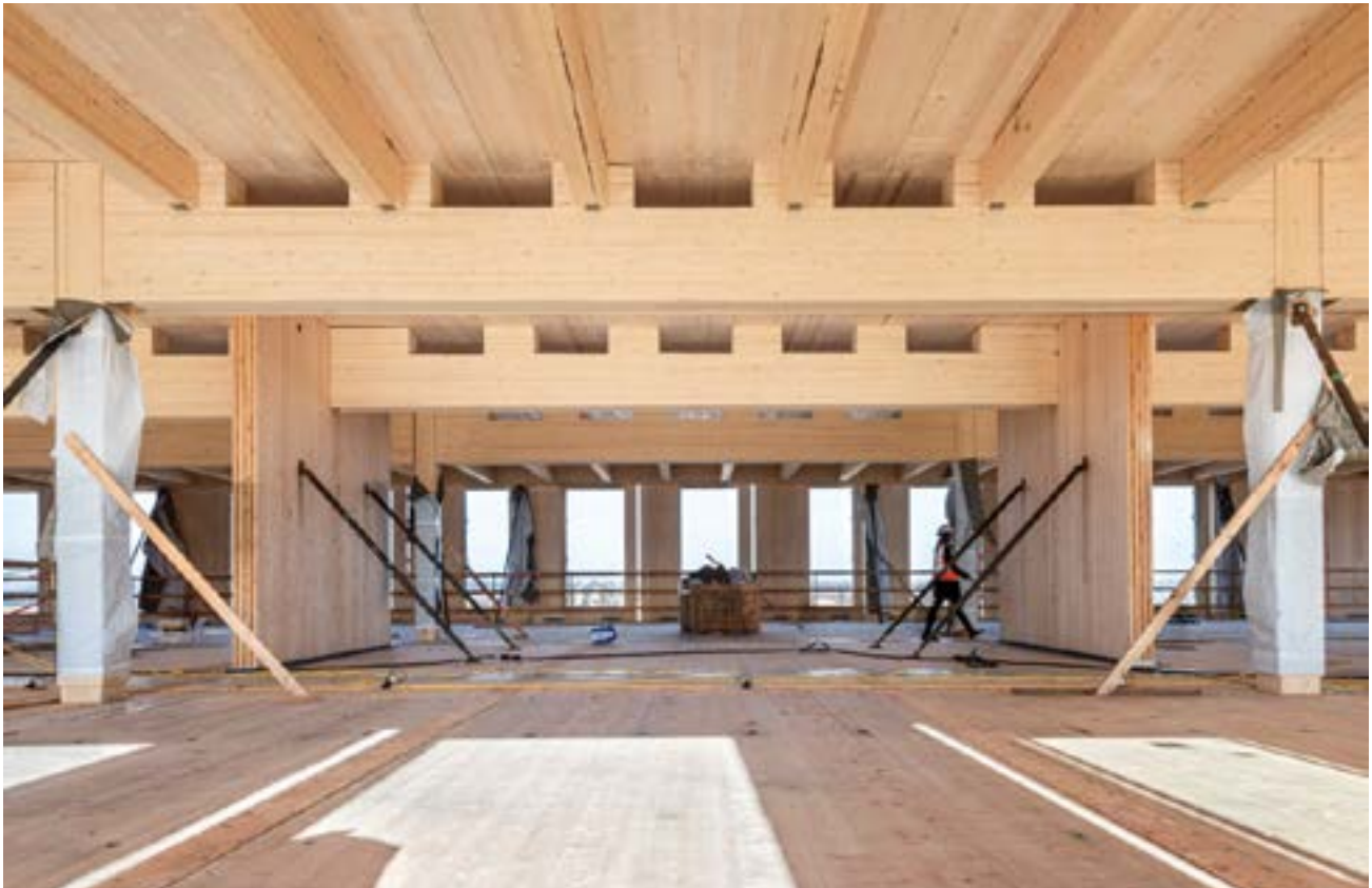
FIGURE 5.19: CATALYST EXAMPLE OF TIMBER-TIMBER COMPOSITE FLOOR PANEL
