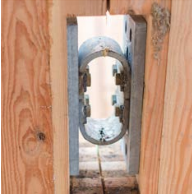
FIGURE 8.10: ROCKING SHEAR WALL FUSE
