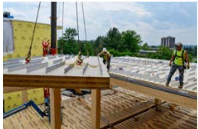
FIGURE 5.16: UMASS AMHERST: EXAMPLE OF COMPOSITE CONCRETE-TIMBER SLABS
