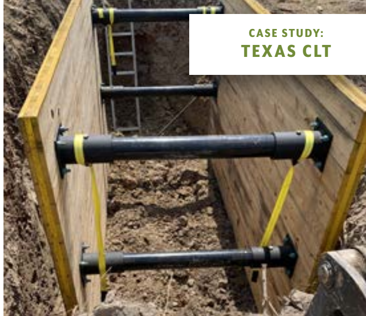
FIGURE 4.5: SHORING USING I-BEAMS AND A MTP
