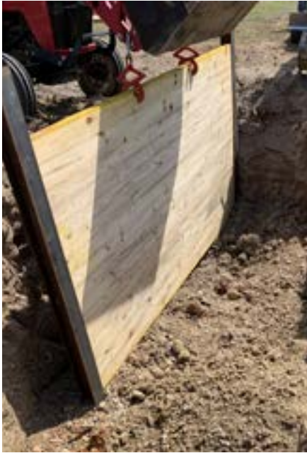
FIGURE 4.4: MASS TIMBER SHORING
