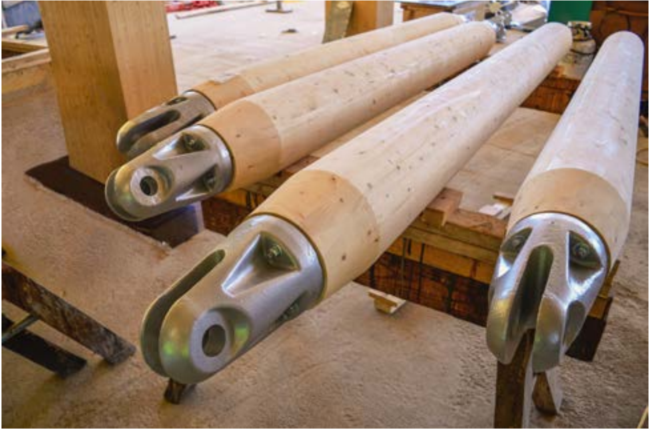
FIGURE 5.13 OFF-THE-SHELF STRUCTURAL METAL CAST COLUMN CONNECTIONS
