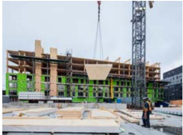
FIGURE 6.13: MASS TIMBER MATERIALS HANDLING
