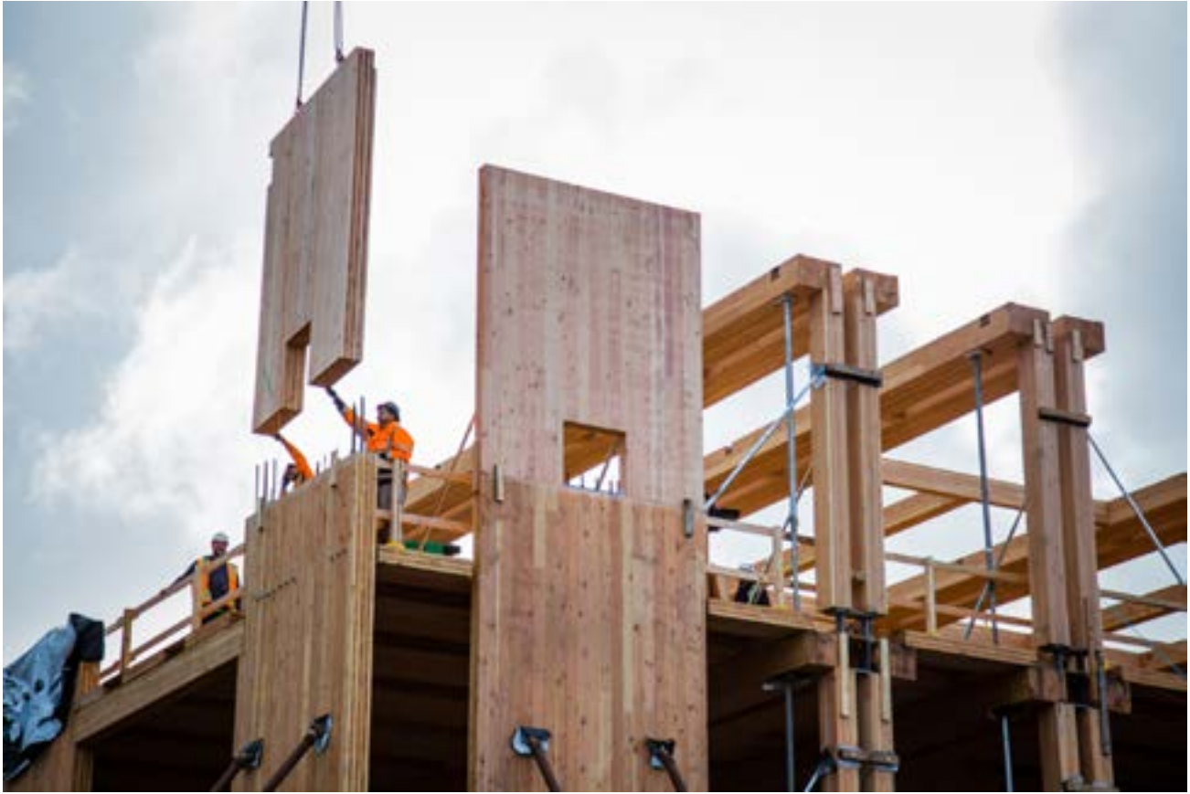
FIGURE 5.21: POST-TENSIONED CLT ‘ROCKING’ SHEAR WALL INSTALLATION
