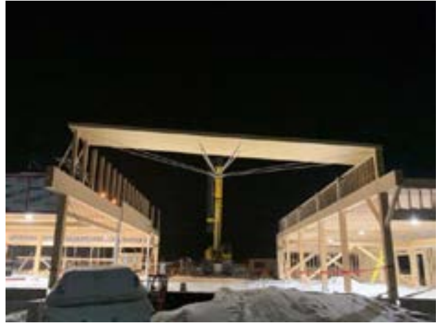
FIGURE 5.18: POST-TENSIONED CLT AT CHIBOUGAMAU TERMINAL IN QUEBEC
