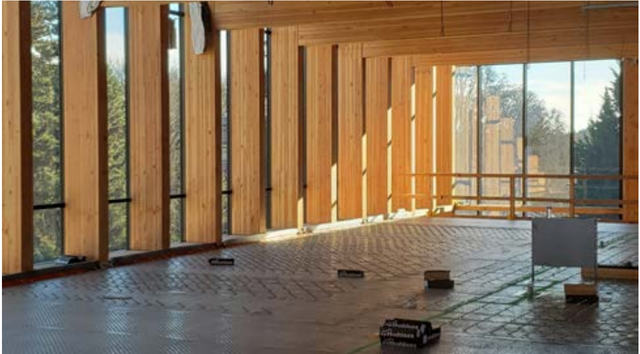
FIGURE 5.15: PEAVY HALL: EXAMPLE OF COMPOSITE CONCRETE-TIMBER SLABS
