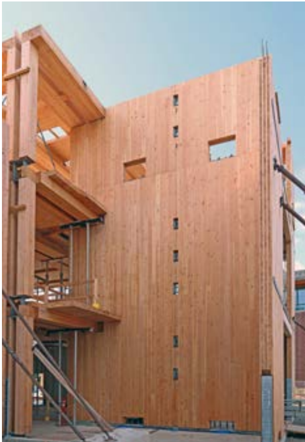
FIGURE 8.9: CLT ROCKING SHEAR WALL WITH STEEL FUSES FOR DISSIPATING SEISMIC FORCES. BROKEN FUSES ARE EASILY REPLACED.
