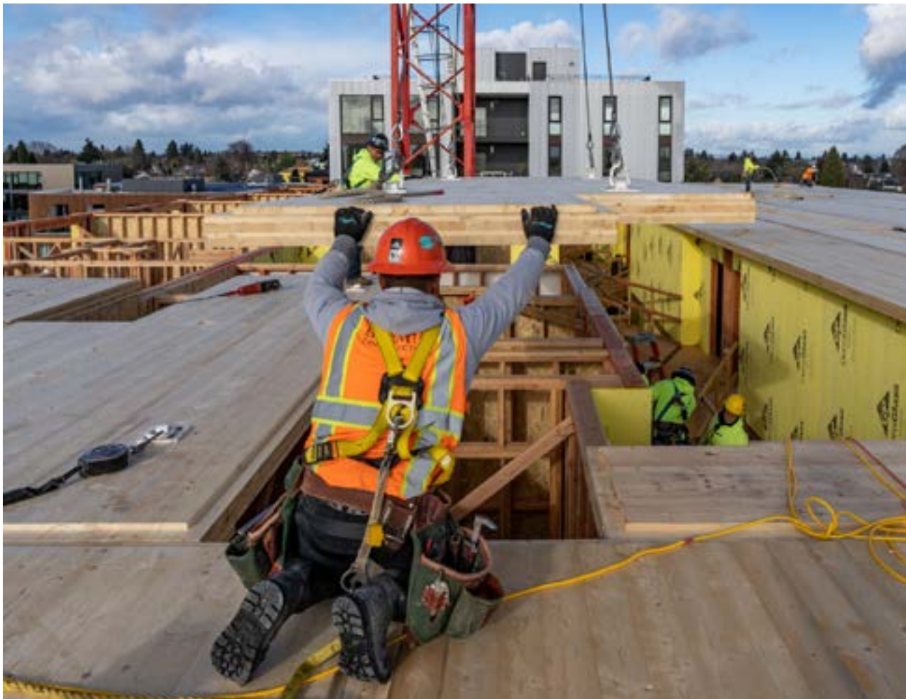
FIGURE 6.7: A SMALL FRAMING CREW GUIDES PANEL PLACEMENT
