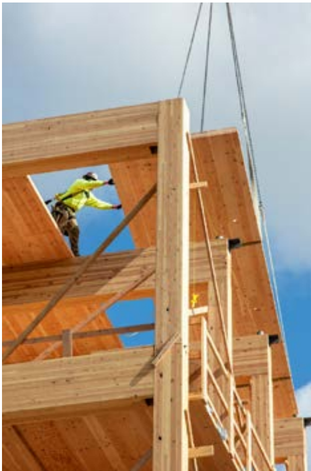
FIGURE 6.15: CLT PANEL ON TIMBER FRAME CRANE INSTALLATION
