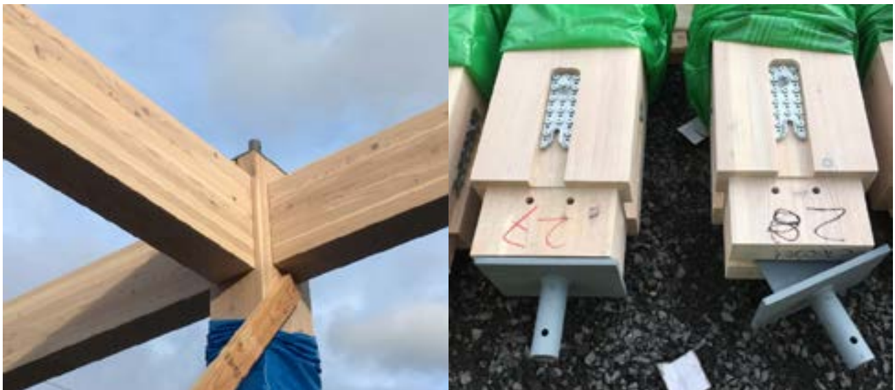
TOP — FIGURE 6.8: OFF-THE-SHELF BEAM CONNECTIONS AND CUSTOM COLUMN CONNECTIONS
