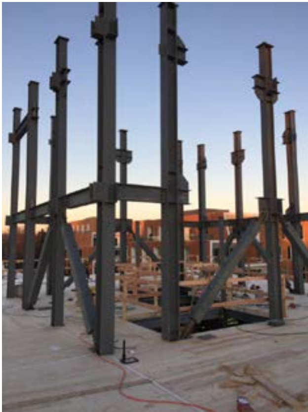
FIGURE 5.20: CLT POST AND BEAM STRUCTURE WITH BUCKLING RESTRAINED BRACED FRAME CORE
