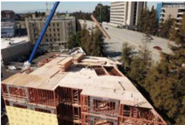
FIGURE 6.5: PRECISION COMPONENTS QUICKLY ASSEMBLED ON A CONSTRAINED SITE
