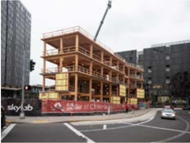
FIGURE 6.14: MODULAR TIMBER CONSTRUCTION ON CONSTRAINED URBAN SITES
