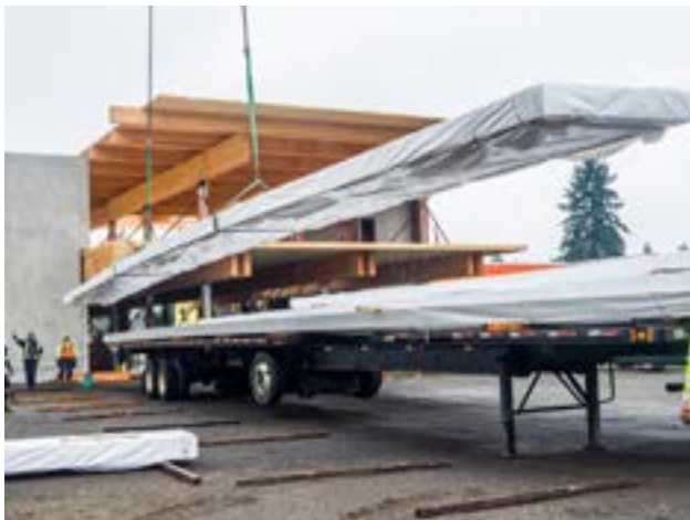
FIGURE 6.19: CLT PANELS PROTECTED WITH WRAP FOR TRANSPORT AND ON-SITE STORAGE
