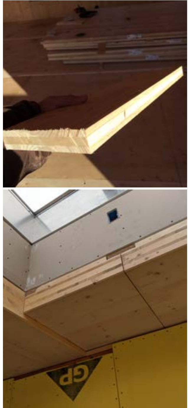
FIGURE 5.11: SPLINE CONNECTION MATERIAL EXAMPLES: JOINERY BOARD AND PLYWOOD
