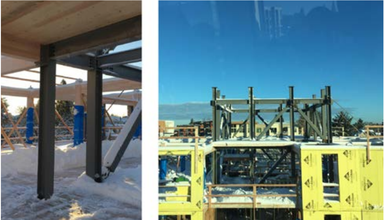
FIGURE 6.17: TIMBER FRAME AND STEEL CORE PROGRESSING IN COLD, SNOWY WEATHER
