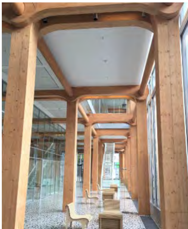
FIGURE 5.9: CNC JOINERY WITH PREFABRICATED MASS TIMBER COLUMNS AND BEAMS
