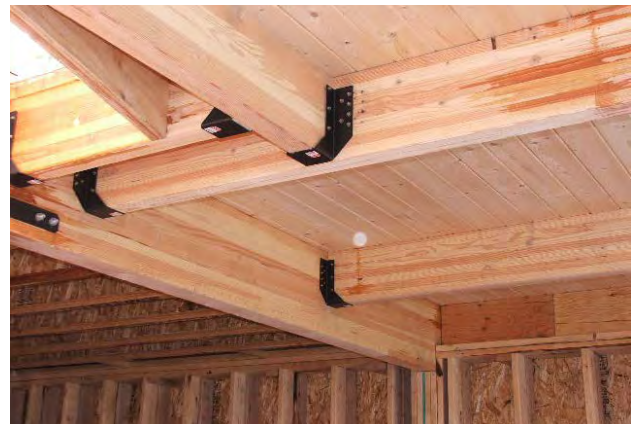
FIGURE 5.8: MASS TIMBER CONNECTOR EXAMPLES
