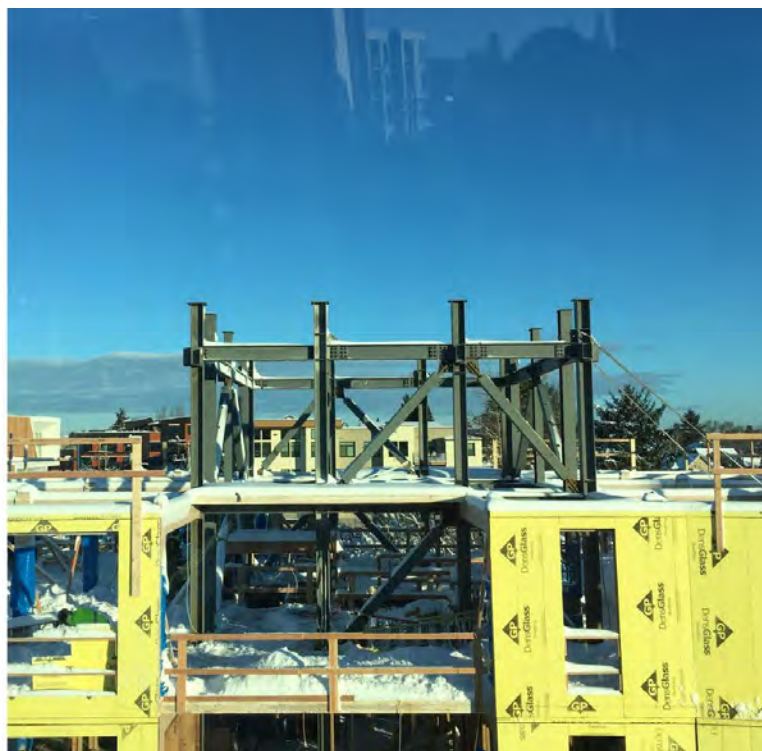
FIGURE 6.17: TIMBER FRAME AND STEEL CORE PROGRESSING IN COLD, SNOWY WEATHER
