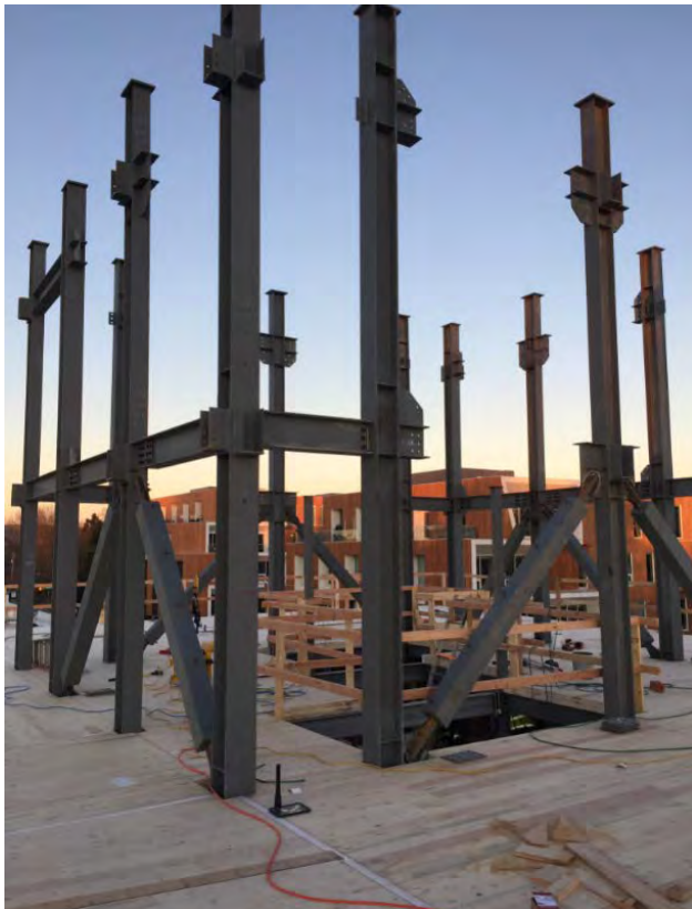
FIGURE 5.23: CLT POST AND BEAM STRUCTURE WITH BUCKLING RESTRAINED BRACED FRAME CORE
