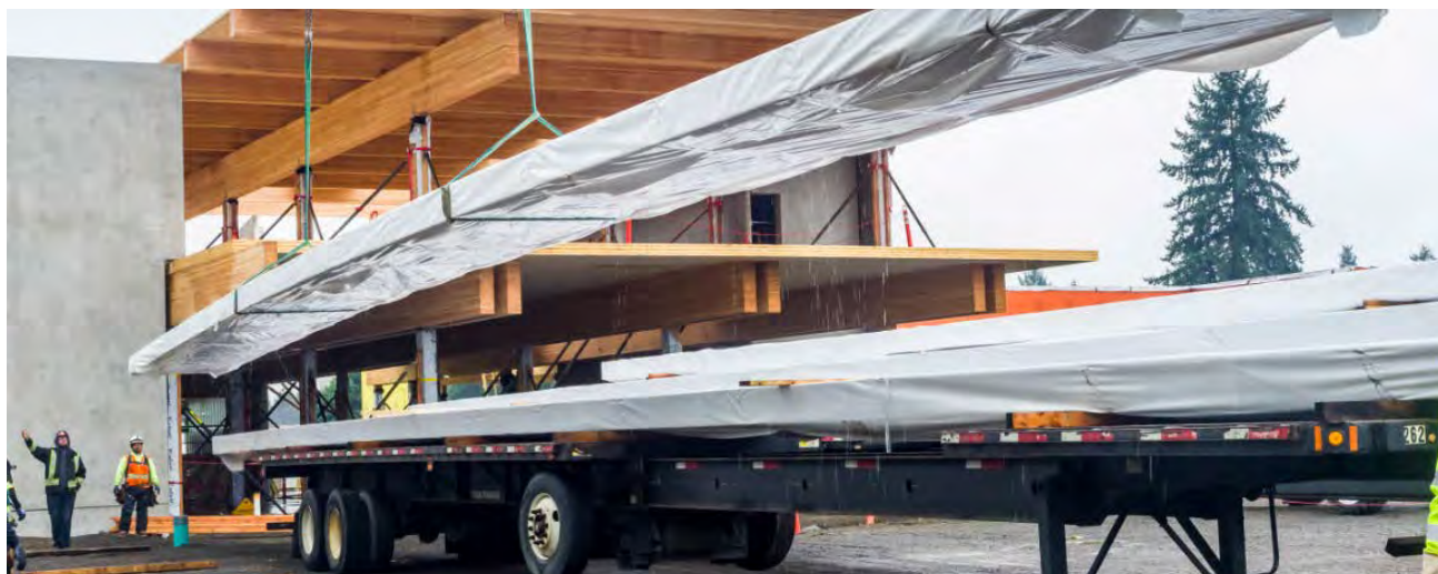
FIGURE 6.19: CLT PANELS PROTECTED WITH WRAP FOR TRANSPORT AND ON-SITE STORAGE
