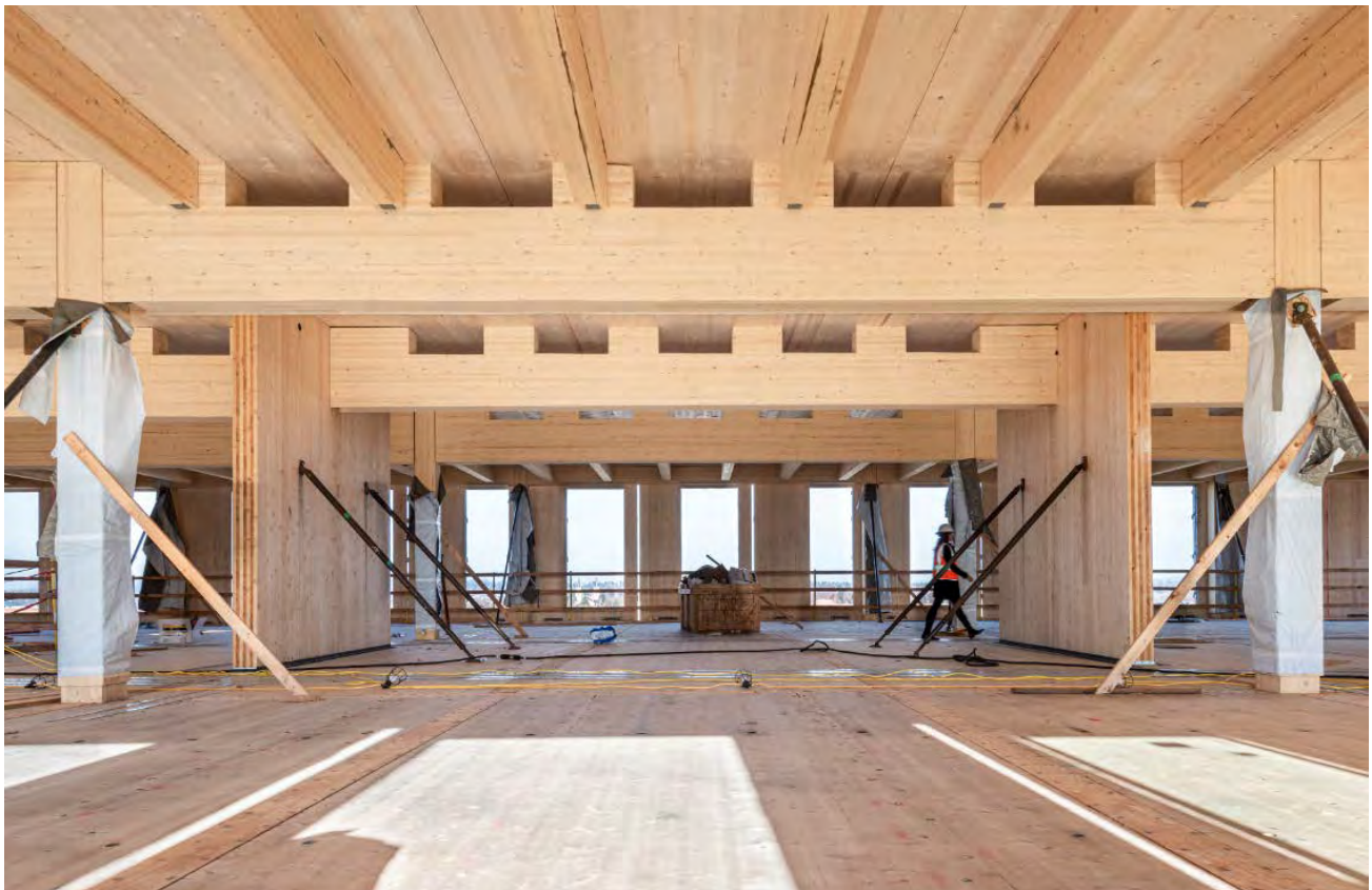
TOP LEFT — FIGURE 5.19: POST TENSIONED TIMBER BEAM
