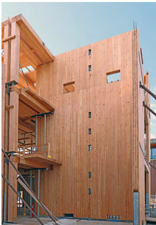
Figure 8.11: CLT Rocking Shear Wall
