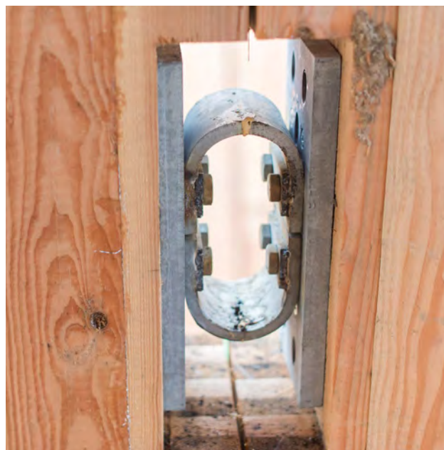
FIGURE 8.12: ROCKING SHEAR WALL FUSE
