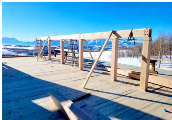
A COMBINATION TIMBER FRAME AND ICLT STRUCTURE DURING CONSTRUCTION Source: Euclid Timber Frame Systems
