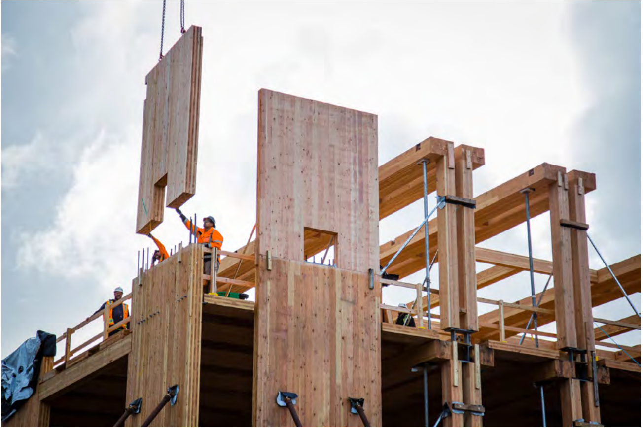
FIGURE 5.25: POST-TENSIONED CLT ‘ROCKING’ SHEAR WALL INSTALLATION
