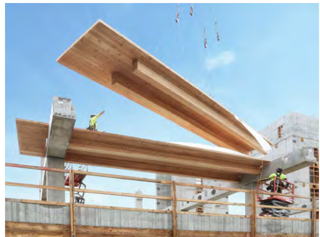
ABOVE AND RIGHT — FIGURE 6.8: COMPOSITE TIMBER AND PRECAST CONCRETE STRUCTURE
