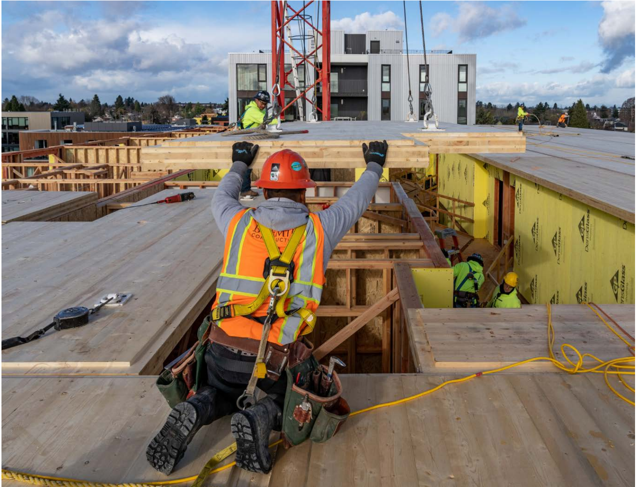
FIGURE 6.7: A SMALL FRAMING CREW GUIDES PANEL PLACEMENT
