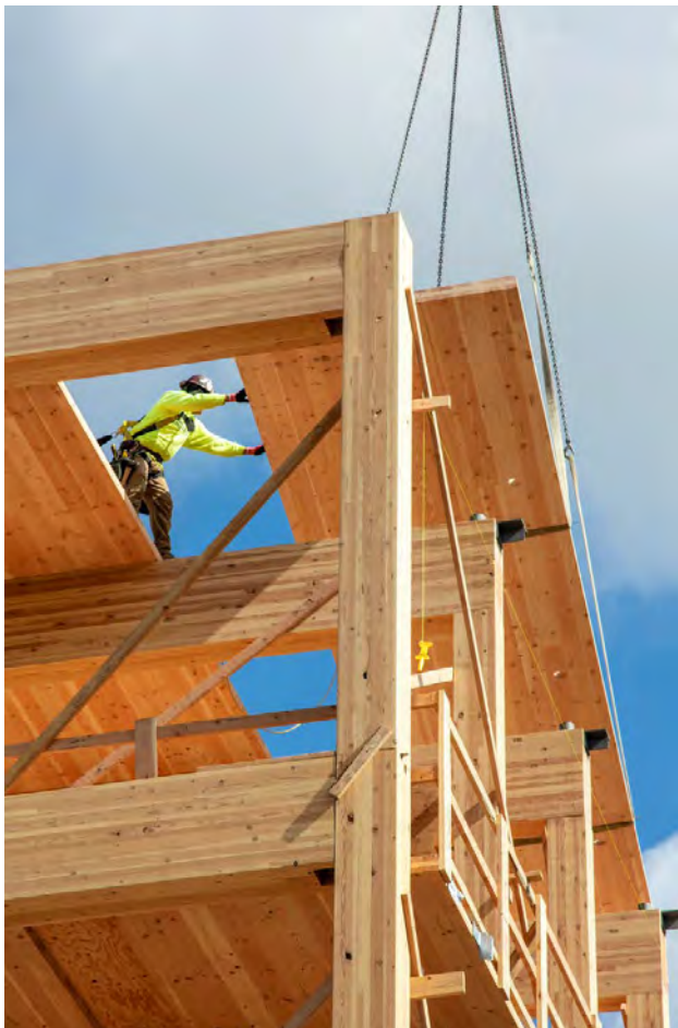
FIGURE 6.15: CRANE LIFTING WITH SLINGS
