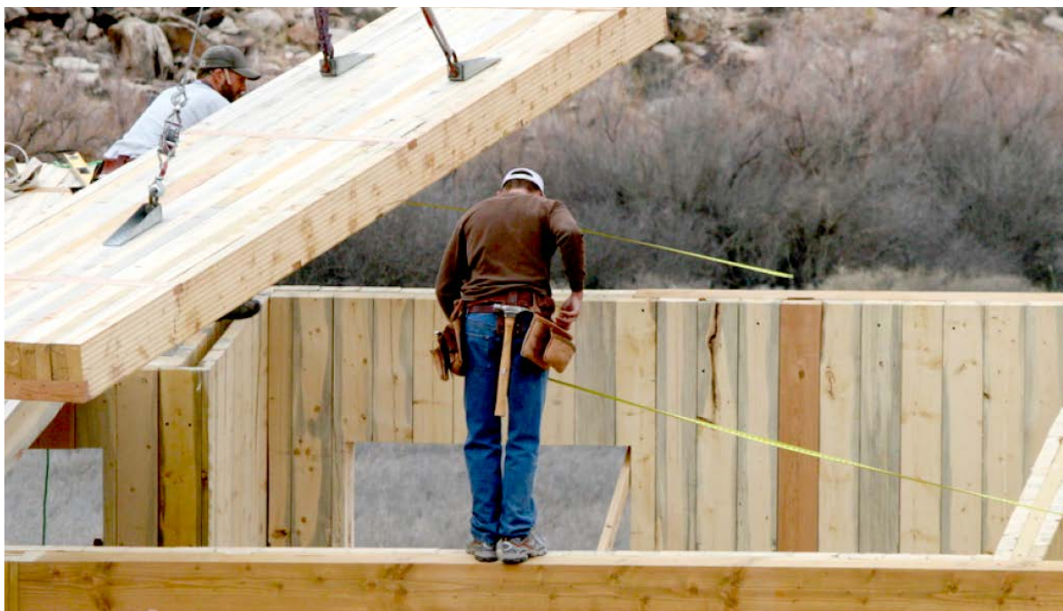
ICLT STRUCTURE DURING CONSTRUCTION
