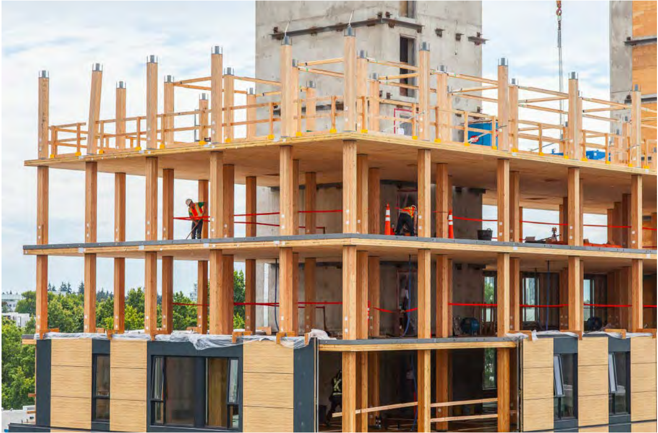
FIGURE 6.4: PREFABRICATED FACADE PANELS FOLLOW CLOSELY BEHIND STRUCTURAL FRAMING
