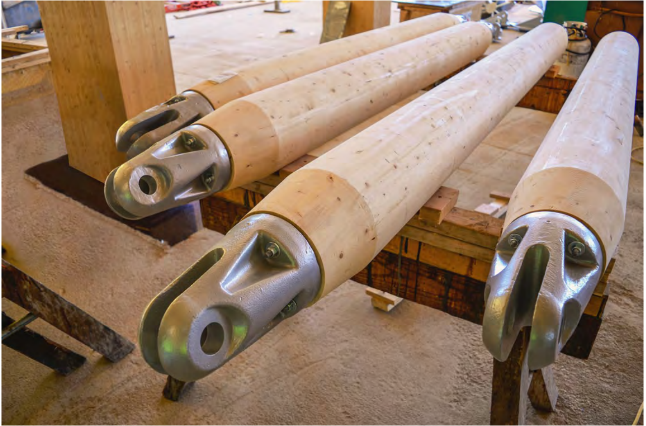
FIGURE 5.13 OFF-THE-SHELF STRUCTURAL METAL CAST COLUMN CONNECTIONS TIMBER END CONNECTORS™, UMASS AMHERST INTEGRATED DESIGN BUILDING
