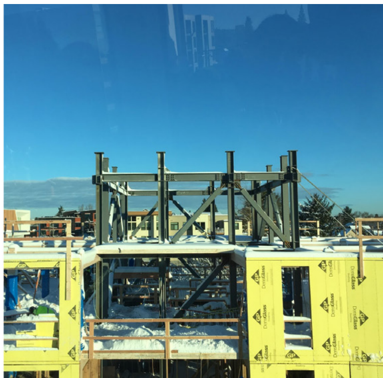
FIGURE 6.19: TIMBER FRAME AND STEEL CORE PROGRESSING IN COLD, SNOWY WEATHER
