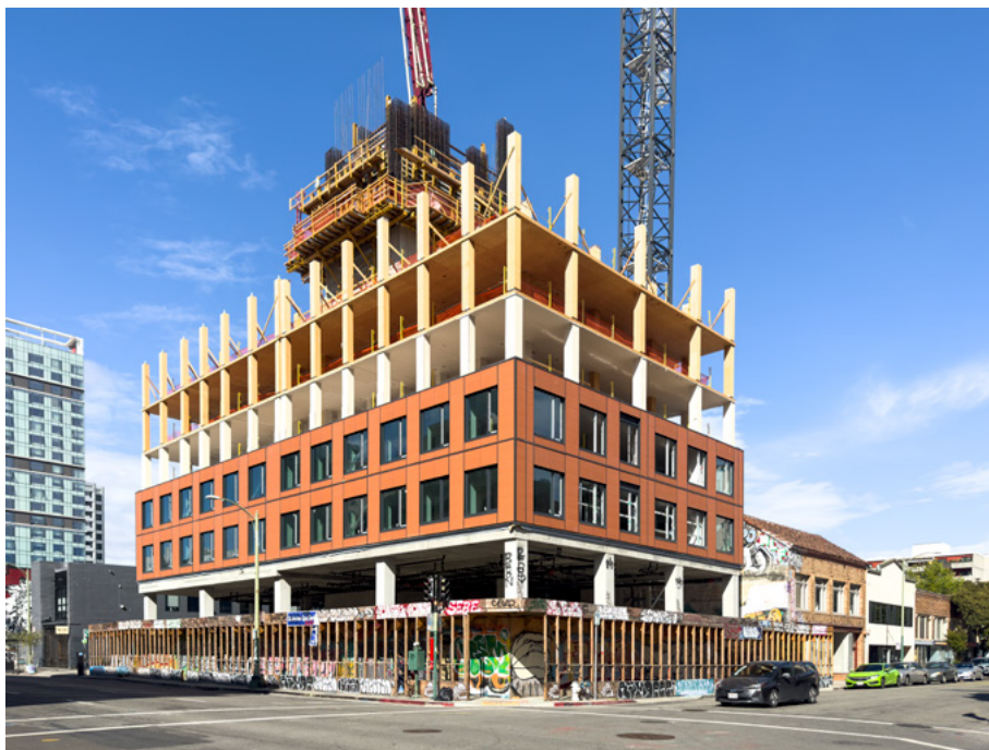
FIGURE 6.5: 25 PERCENT COST SAVINGS WITH MASS TIMBER STRUCTURE AND PREFABRICATED FACADE PANELS
