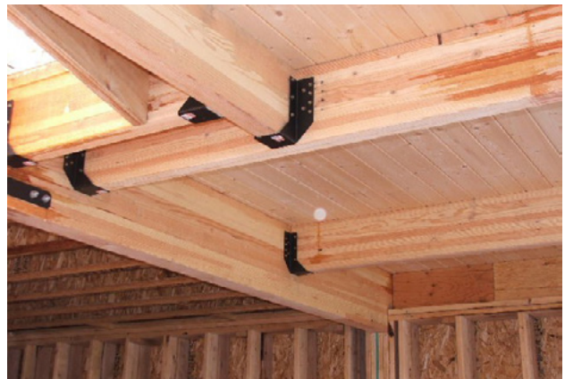
FIGURE 5.4: MASS TIMBER CONNECTOR EXAMPLES
