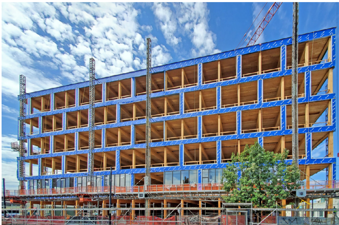
FIGURE 6.20: DISTRICT OFFICE IMPLEMENTED A MOISTURE MANAGEMENT PLAN
