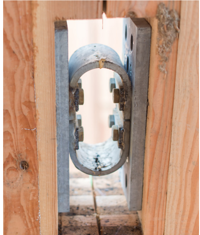
FIGURE 8.19: ROCKING SHEAR WALL FUSE
