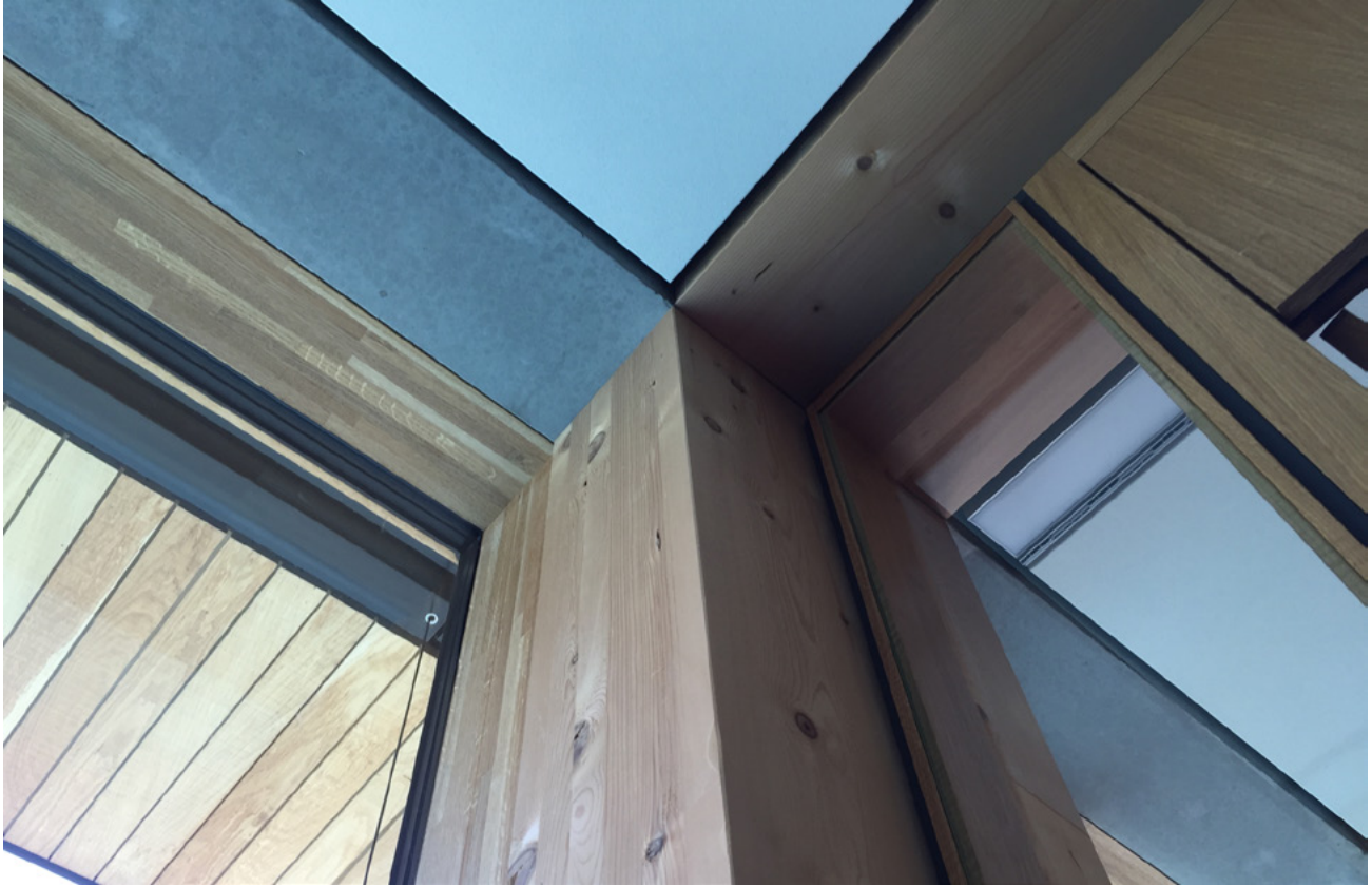
FIGURE 5.32: PRECISE PREFABRICATED MATERIAL INTERSECTIONS
