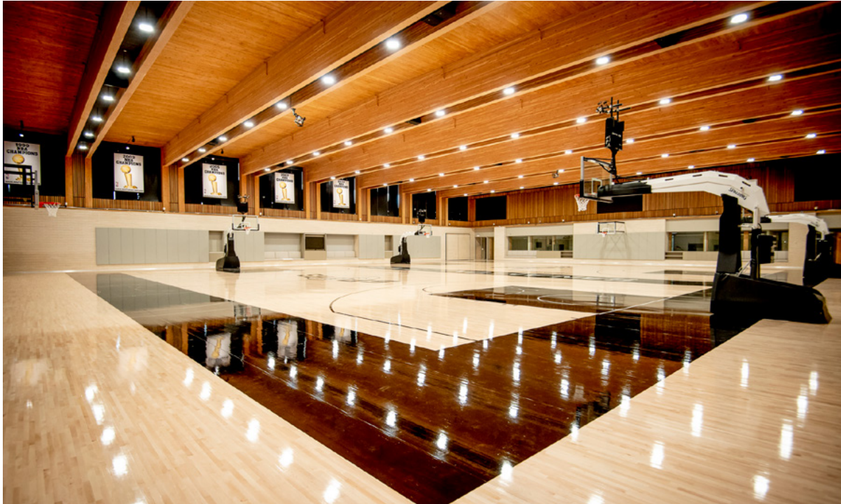
THE BUILDING FEATURES A MASSIVE 130-FOOT CLEAR SPAN.
