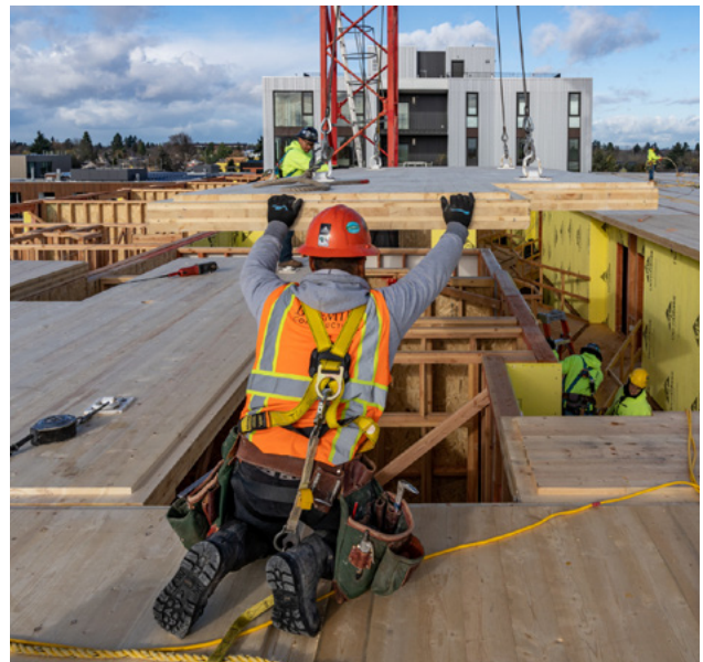
FIGURE 6.10: A SMALL FRAMING CREW GUIDES PANEL PLACEMENT
