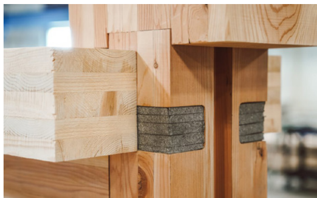
ABOVE — FIGURE 5.5: CNC COLUMN AND BEAM JOINERY
