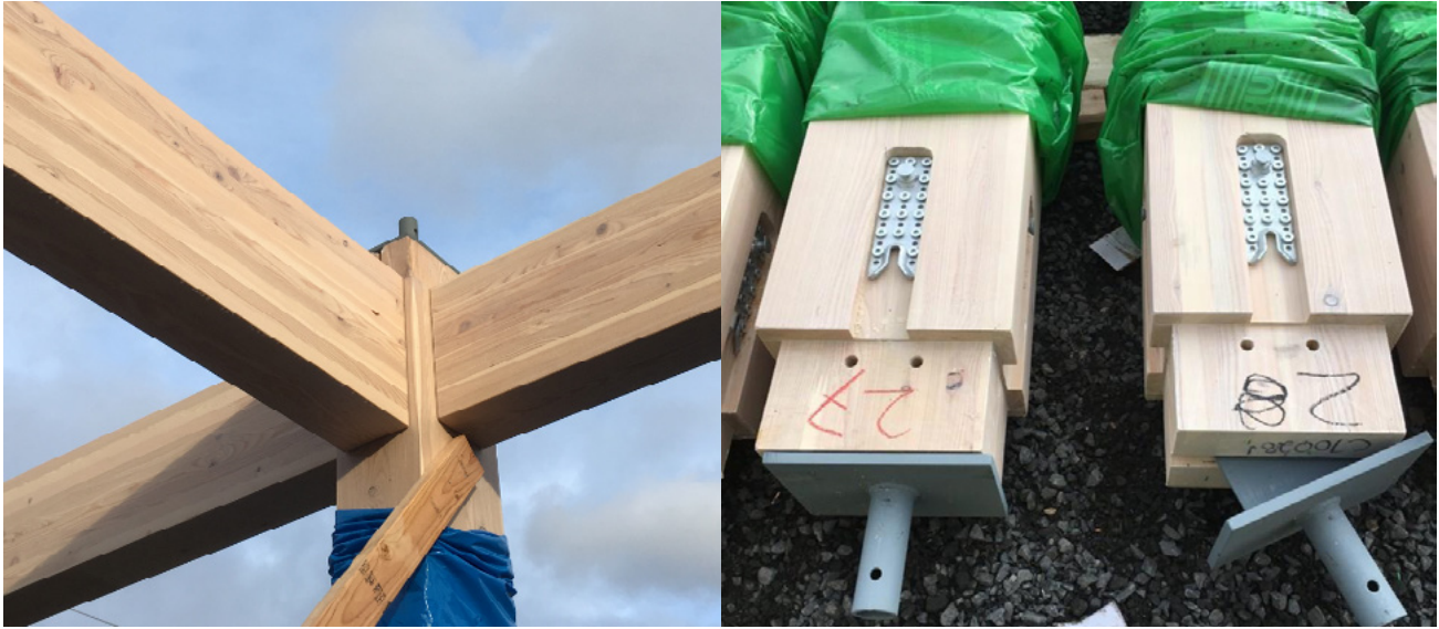
FIGURE 6.14: OFF-THE-SHELF BEAM CONNECTIONS AND CUSTOM COLUMN CONNECTIONS
