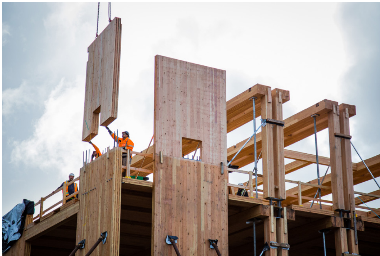
FIGURE 5.25: POST-TENSIONED CLT ‘ROCKING’ SHEAR WALL INSTALLATION
