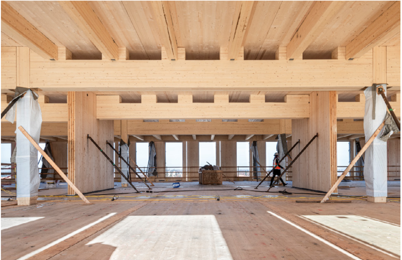
TOP LEFT — FIGURE 5.19: POST-TENSIONED TIMBER BEAM
