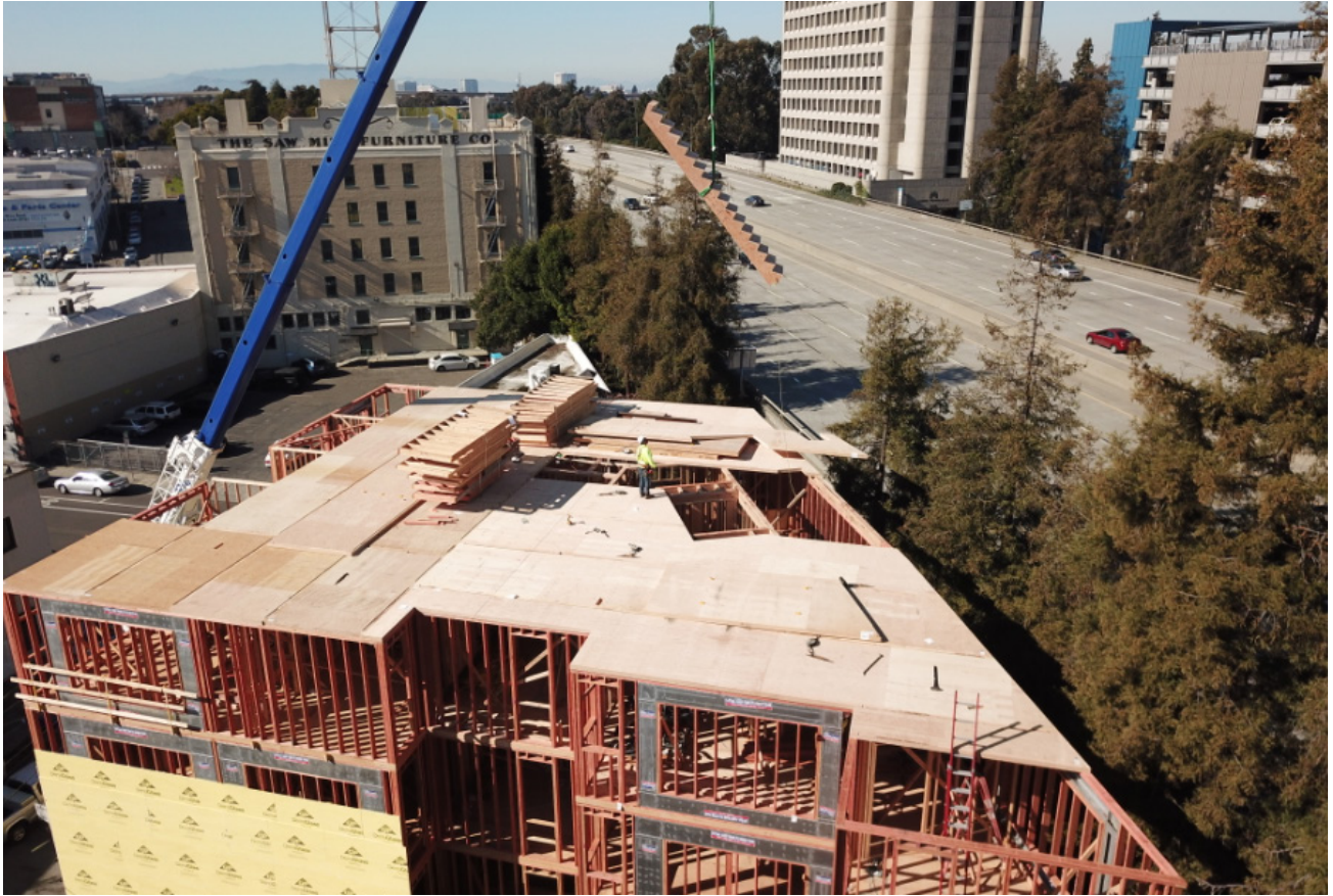
FIGURE 6.7: PRECISION COMPONENTS QUICKLY ASSEMBLED ON A CONSTRAINED SITE
