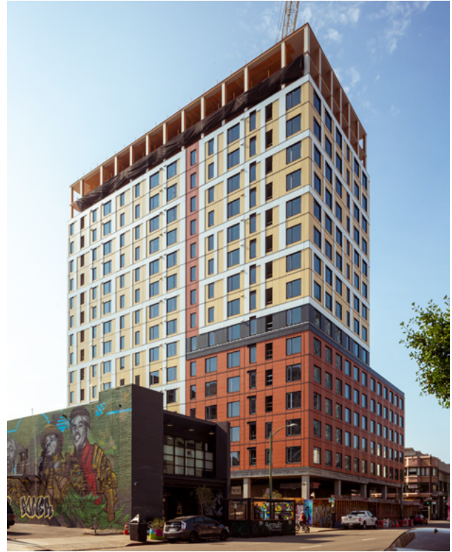
FIGURE 5.39: ONE STORY OF STEEL OVER 16 STORES OF TYPE IV-A OVER
