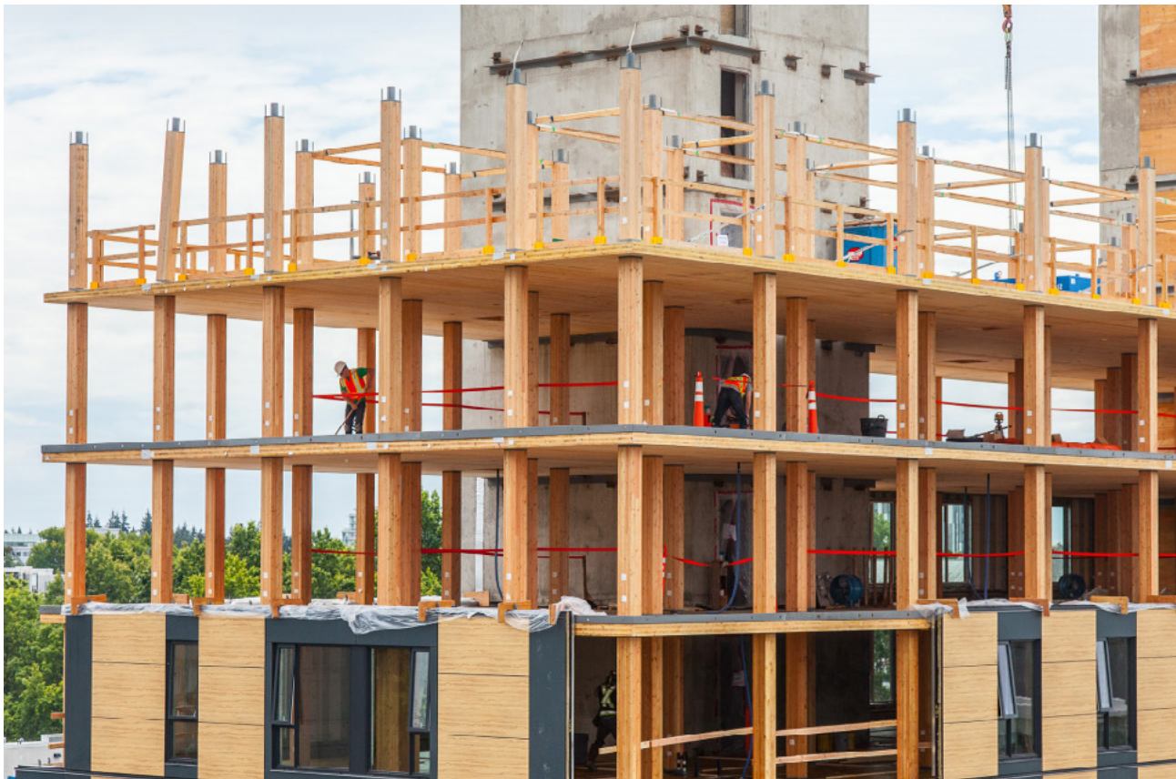
FIGURE 6.8: PREFABRICATED FACADE PANELS FOLLOW CLOSELY BEHIND STRUCTURAL FRAMING
