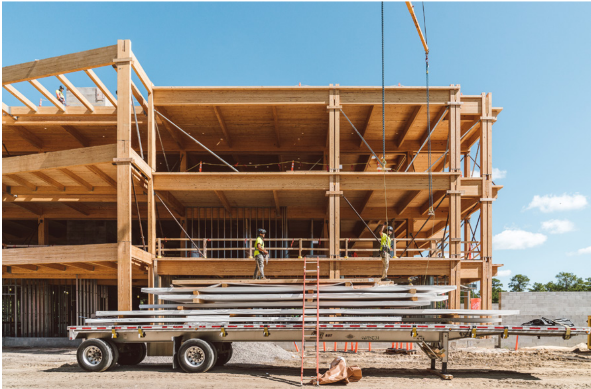
MASS TIMBER DELIVERY AND INSTALLATION
