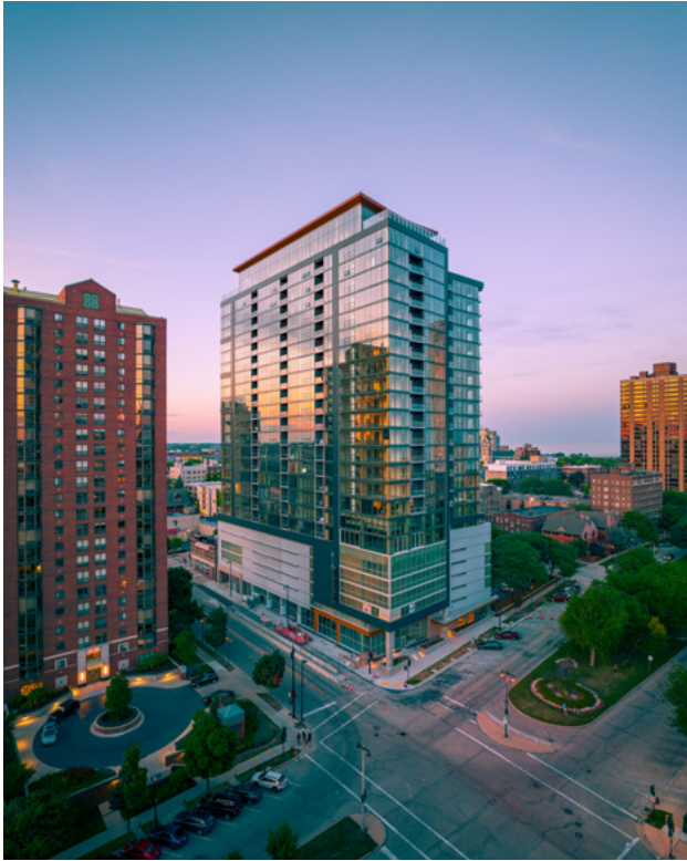
FIGURE 5.38: 19 STORIES TYPE IV-HT OVER A 6-STORY CONCRETE PODIUM
