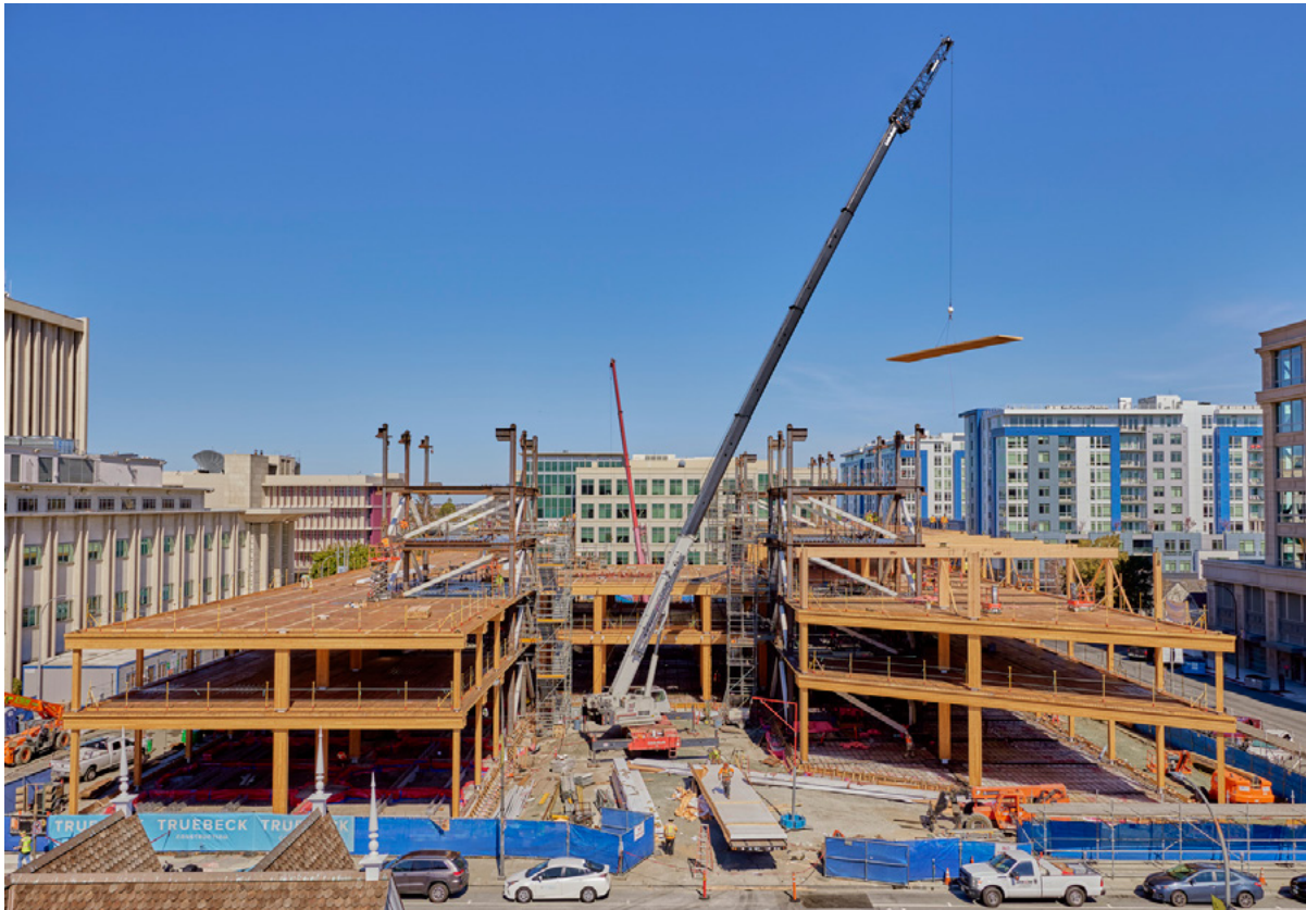
THE MASS TIMBER FRAME IS ERECTED AT SAN MATEO COUNTY'S COB3.
