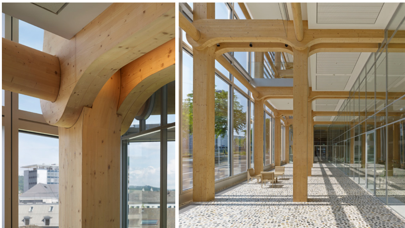
ABOVE — FIGURE 5.5: CNC COLUMN AND BEAM JOINERY
