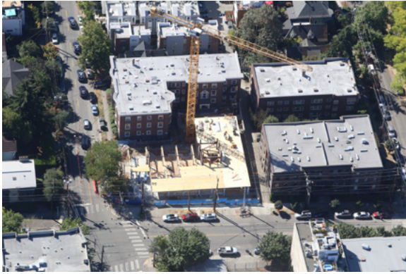
HEARTWOOD IS A WORKFORCE HOUSING DEVELOPMENT IN SEATTLE. THE TYPE IV-C PROJECT CAPITALIZED ON A MASS TIMBER/STEEL HYBRID SYSTEM AND CUSTOM MORTISE-AND-TENON BEAM CONNECTION TO ACHIEVE ITS SEISMIC AND FIRE RATING PERFORMANCE STANDARDS.
