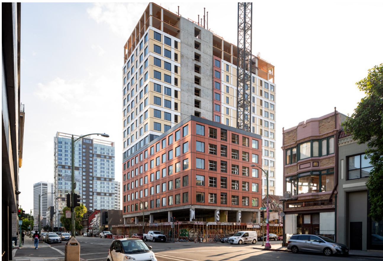
FIGURE 8.9: 19-STORY MPP TOWER SAVED OVER 25% ON COSTS AND 6 MONTHS OF CONSTRUCTION TIME.
