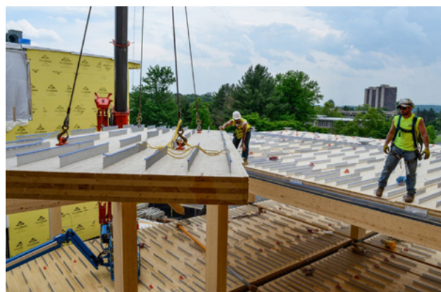
TOP – FIGURE 5.17: COMPOSITE CONCRETE-TIMBER SLAB WITH ACOUSTIC MAT AND INCLINED SCREW REINFORCING
