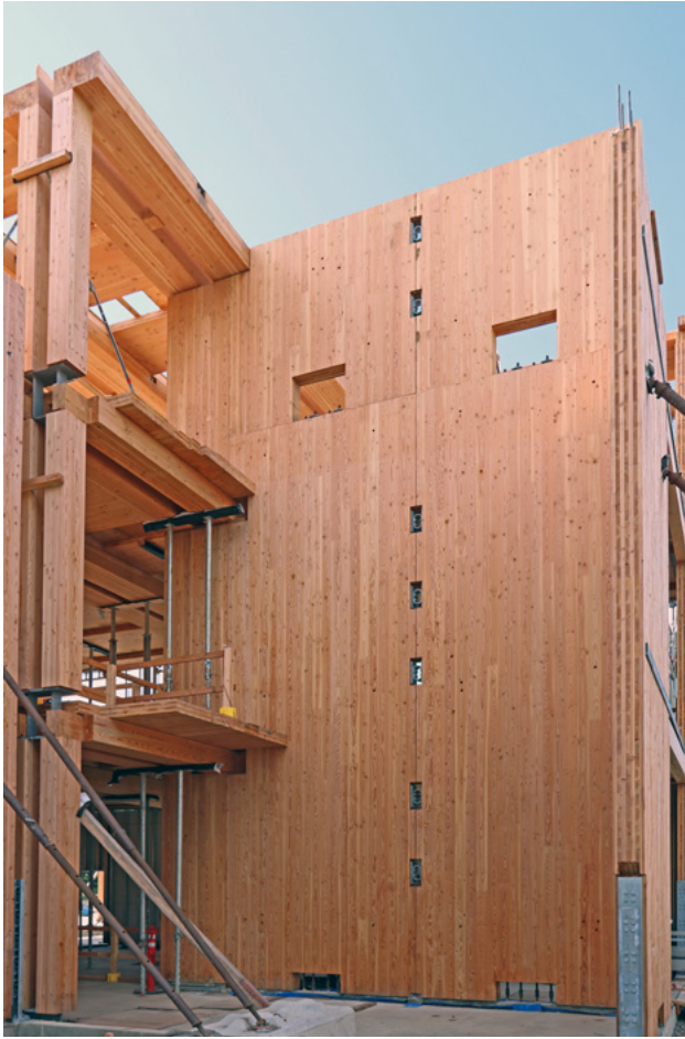
FIGURE 8.18: CLT ROCKING SHEAR WALL
