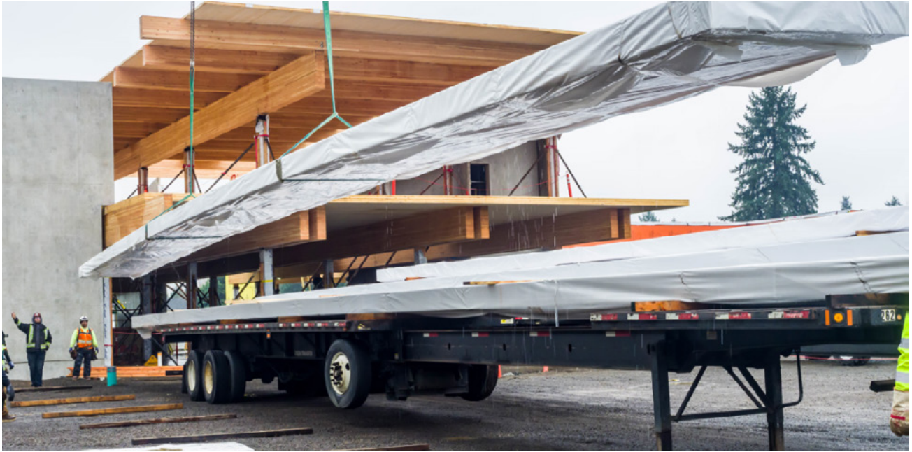
FIGURE 6.21: CLT PANELS PROTECTED WITH WRAP FOR TRANSPORT AND ON-SITE STORAGE
