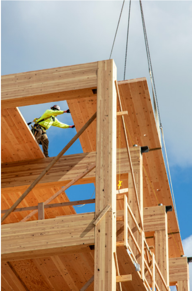
FIGURE 6.17: CRANE LIFTING WITH SLINGS
