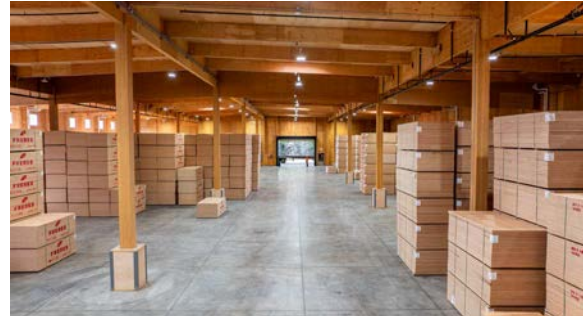
THE WAREHOUSE FEATURES A 40-FOOT-BY-48-FOOT GRID
