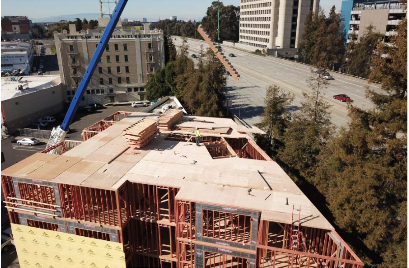
FIGURE 6.9: PRECISION COMPONENTS QUICKLY ASSEMBLED ON A CONSTRAINED SITE
