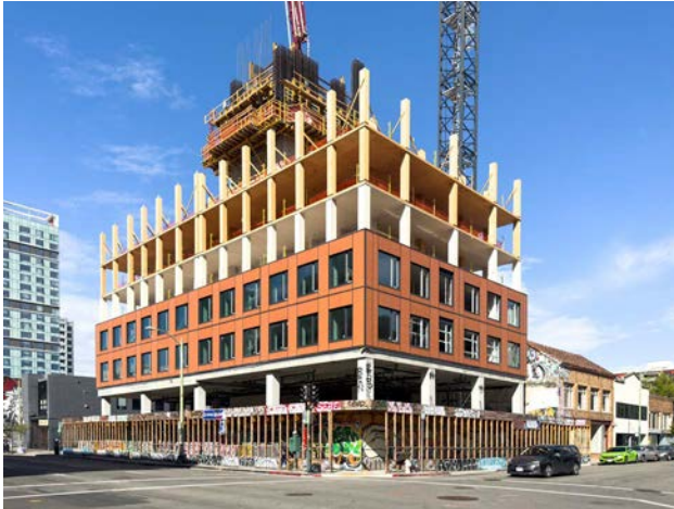
FIGURE 6.6: MASS TIMBER STRUCTURE AND PREFABRICATED FACADE PANELS
