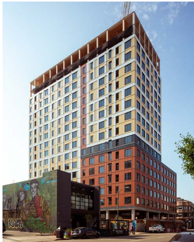
FIGURE 5.39: 1 STORY OF STEEL OVER 16 STORIES OF TYPE IV-A
