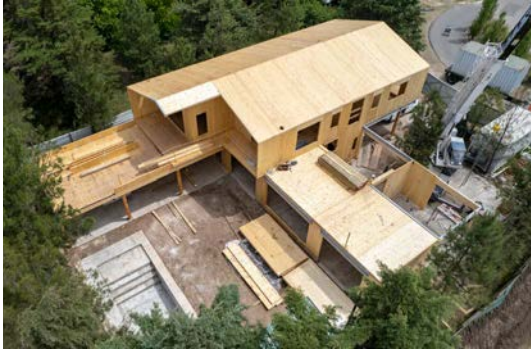
CLT HOUSE SAN NICOLAS UNDER CONSTRUCTION, WITH THE MASS TIMBER STRUCTURE EXPOSED
