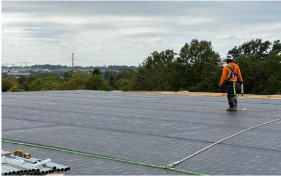
SLOPESHIELD PLUS ADHERED TO 3-PLY CLT PANELS
