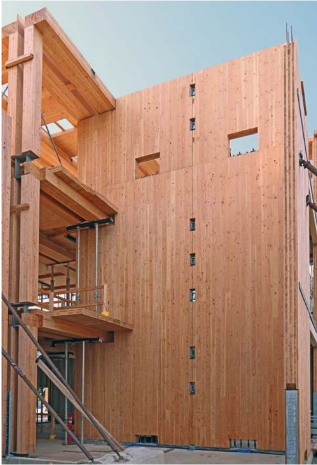
FIGURE 8.18: CLT ROCKING SHEAR WALL
