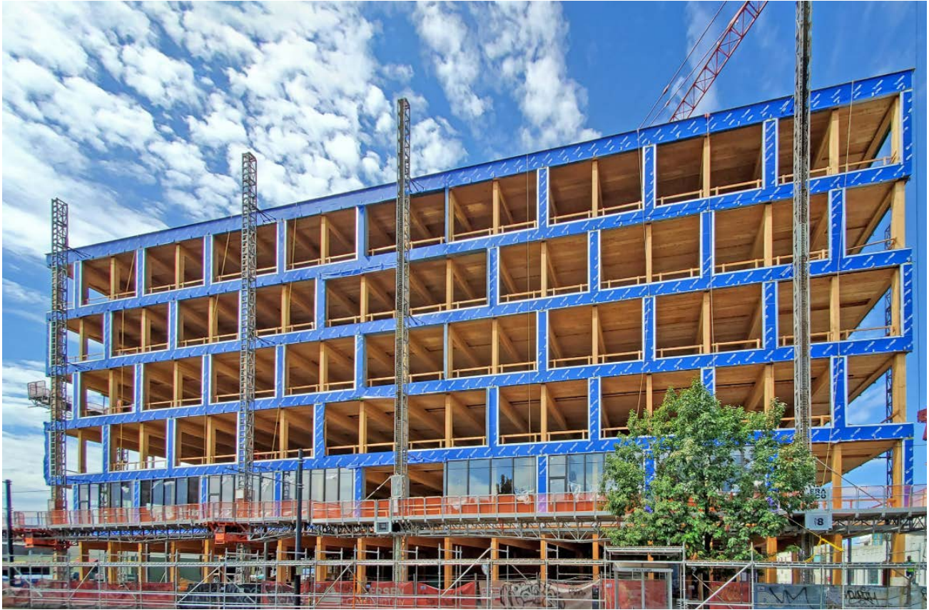
FIGURE 6.22: DISTRICT OFFICE IMPLEMENTED A MOISTURE MANAGEMENT PLAN
