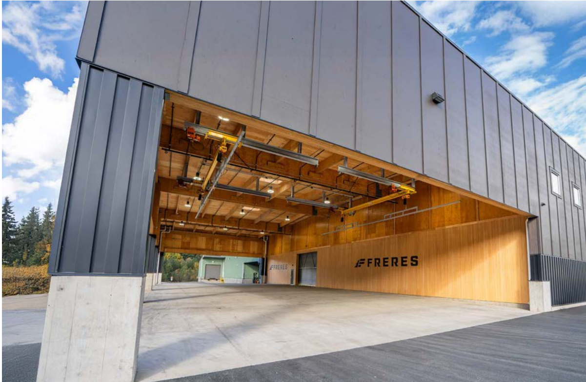
THE 58,000-SQUARE-FOOT MASS TIMBER WAREHOUSE MIMICS TILT-UP CONCRETE CONSTRUCTION
