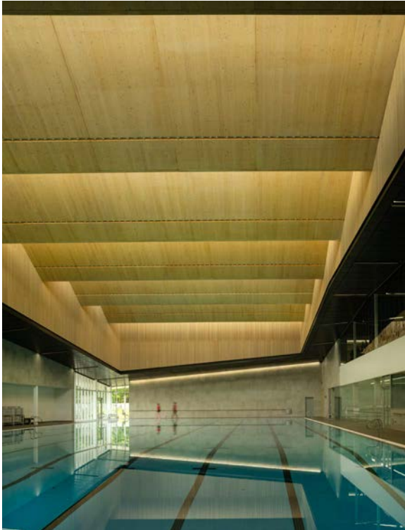
THE 50-METER LAP POOL HAS A MASS TIMBER ROOF IN A SAWTOOTH DESIGN
