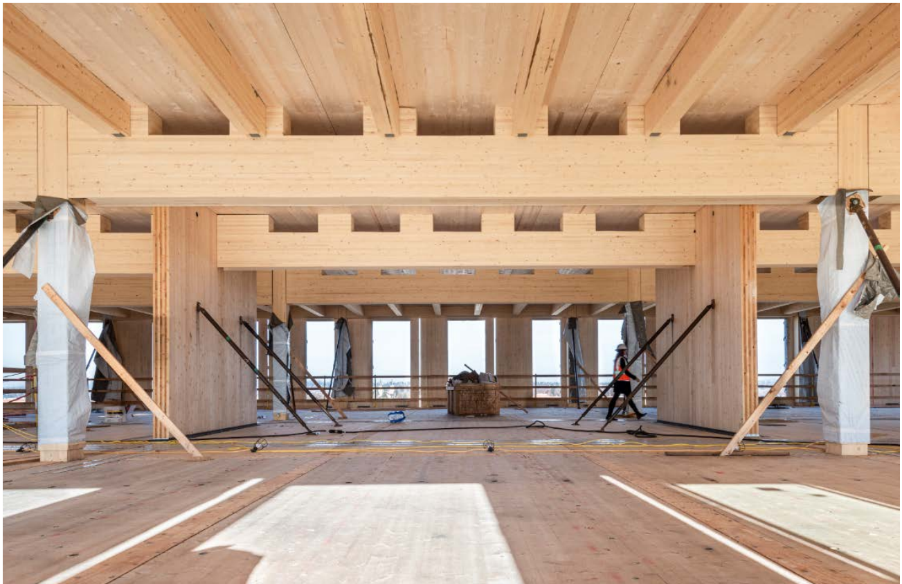
TOP LEFT — FIGURE 5.19: POST-TENSIONED TIMBER BEAM
