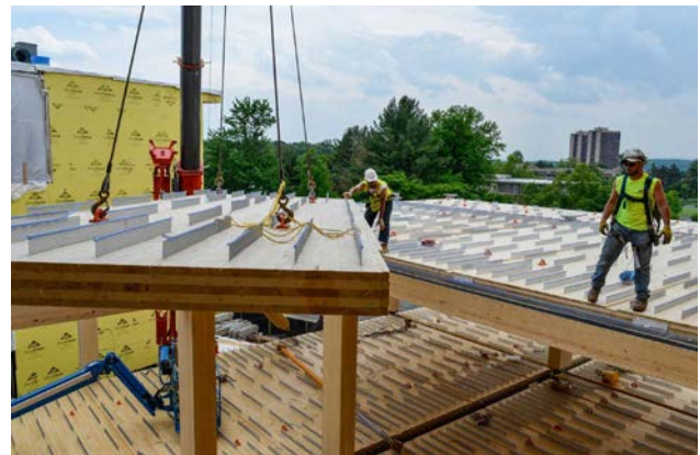
TOP — FIGURE 5.17: COMPOSITE CONCRETE-TIMBER SLAB WITH ACOUSTIC MAT AND INCLINED SCREW REINFORCING
