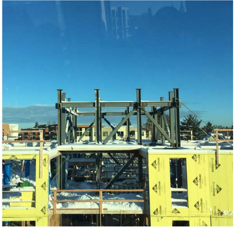
FIGURE 6.21: TIMBER FRAME AND STEEL CORE PROGRESSING IN COLD, SNOWY WEATHER
