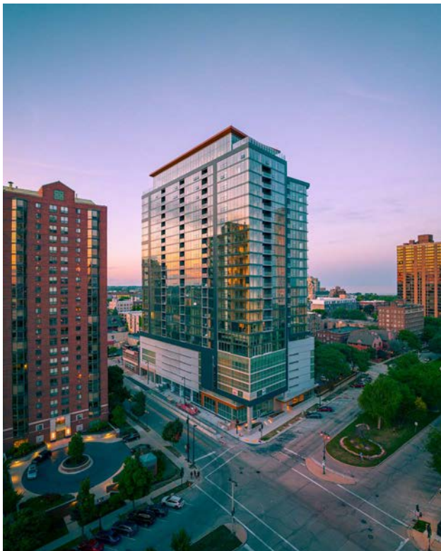
FIGURE 5.38: 19 STORIES TYPE IV-HT OVER A 6-STORY CONCRETE PODIUM
