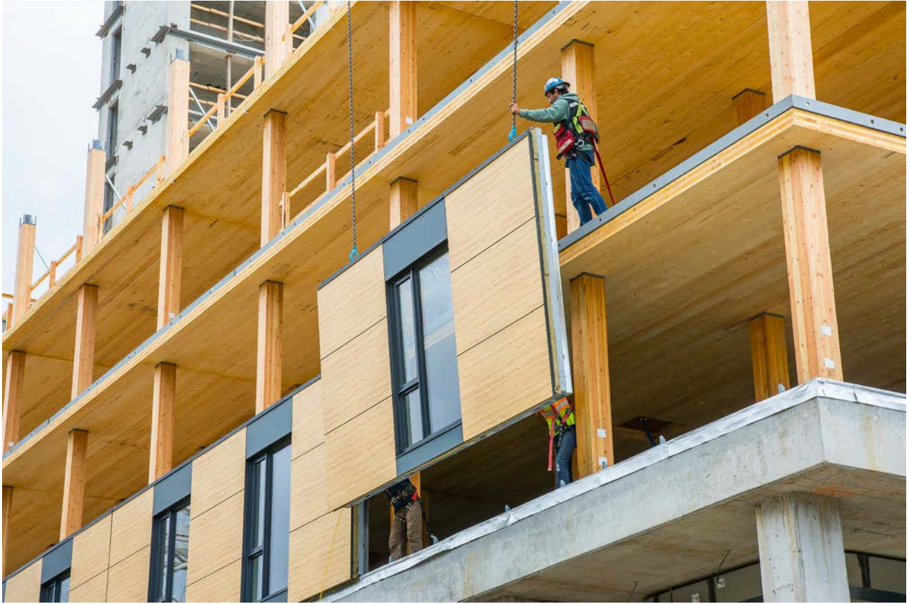
FIGURE 6.10: PREFABRICATED FACADE PANELS FOLLOW CLOSELY BEHIND STRUCTURAL FRAMING
