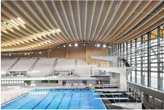
THE CLEARANCE HEIGHT ABOVE THE DIVING PLATFORM IS REFLECTED IN THE UNDULATING GEOMETRY OF THE OLYMPIC AQUATICS CENTRE ROOF Source: © Jad Sylla, for schlaich bergermann partner
