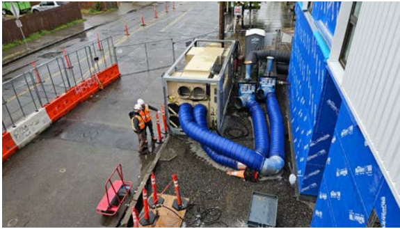
POLYGON CLIMATE CONTROL EQUIPMENT (DESICCANT DEHUMIDIFIER AND INDIRECT FIRED HEATERS) TREAT INTERIOR CONDITIONS OF TIMBERVIEW VIII
