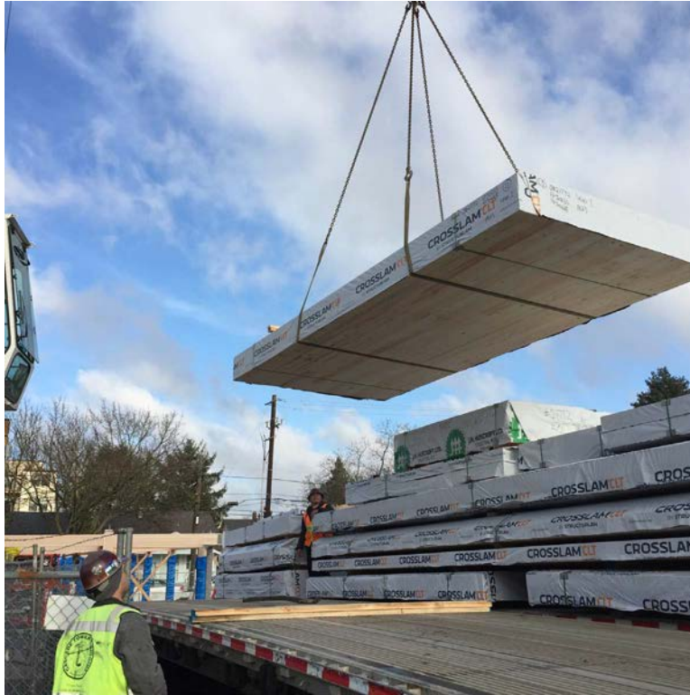
FIGURE 6.24: CLT PANELS PROTECTED WITH WRAP FOR TRANSPORT AND ON-SITE STORAGE
