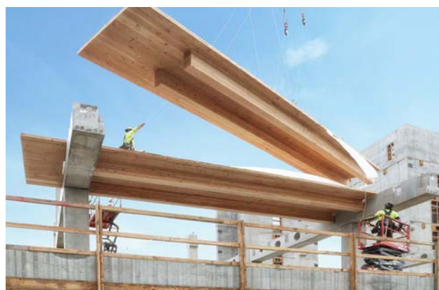
ABOVE AND RIGHT – FIGURE 6.13: COMPOSITE TIMBER AND PRECAST CONCRETE STRUCTURE
