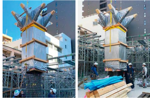
LOWERING PERMANENT CLT FORMWORK OVER STEEL REBAR BY CRANE
