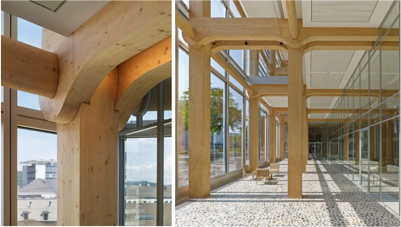
FIGURE 5.5: CNC COLUMN AND BEAM JOINERY
