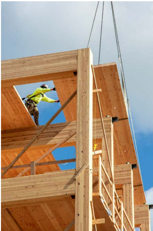
FIGURE 6.19: CRANE LIFTING WITH SLINGS
