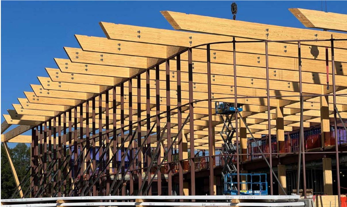
THE BUILDING IS DESIGNED WITH GLULAM POSTS AND BEAMS
