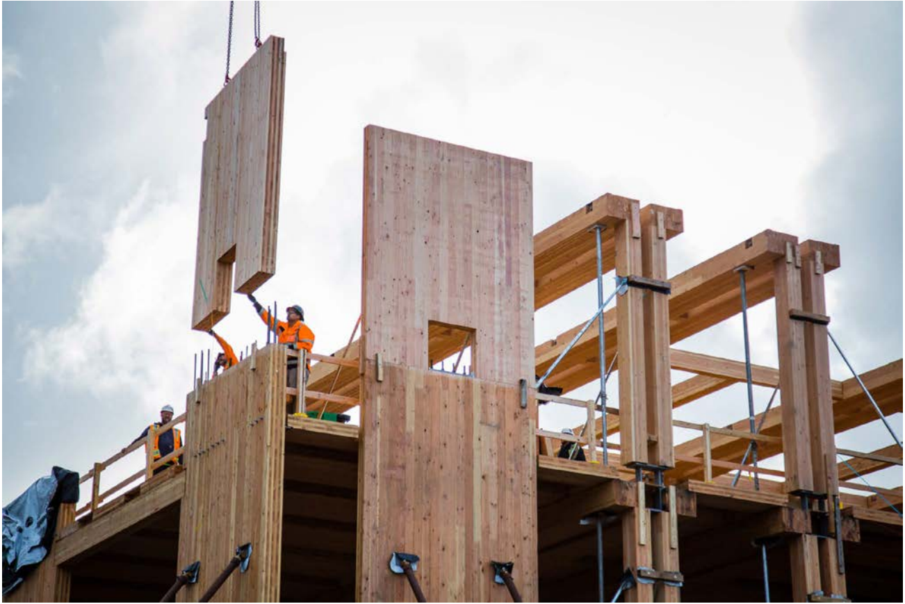
FIGURE 5.25: POST-TENSIONED CLT 'ROCKING' SHEAR WALL INSTALLATION
